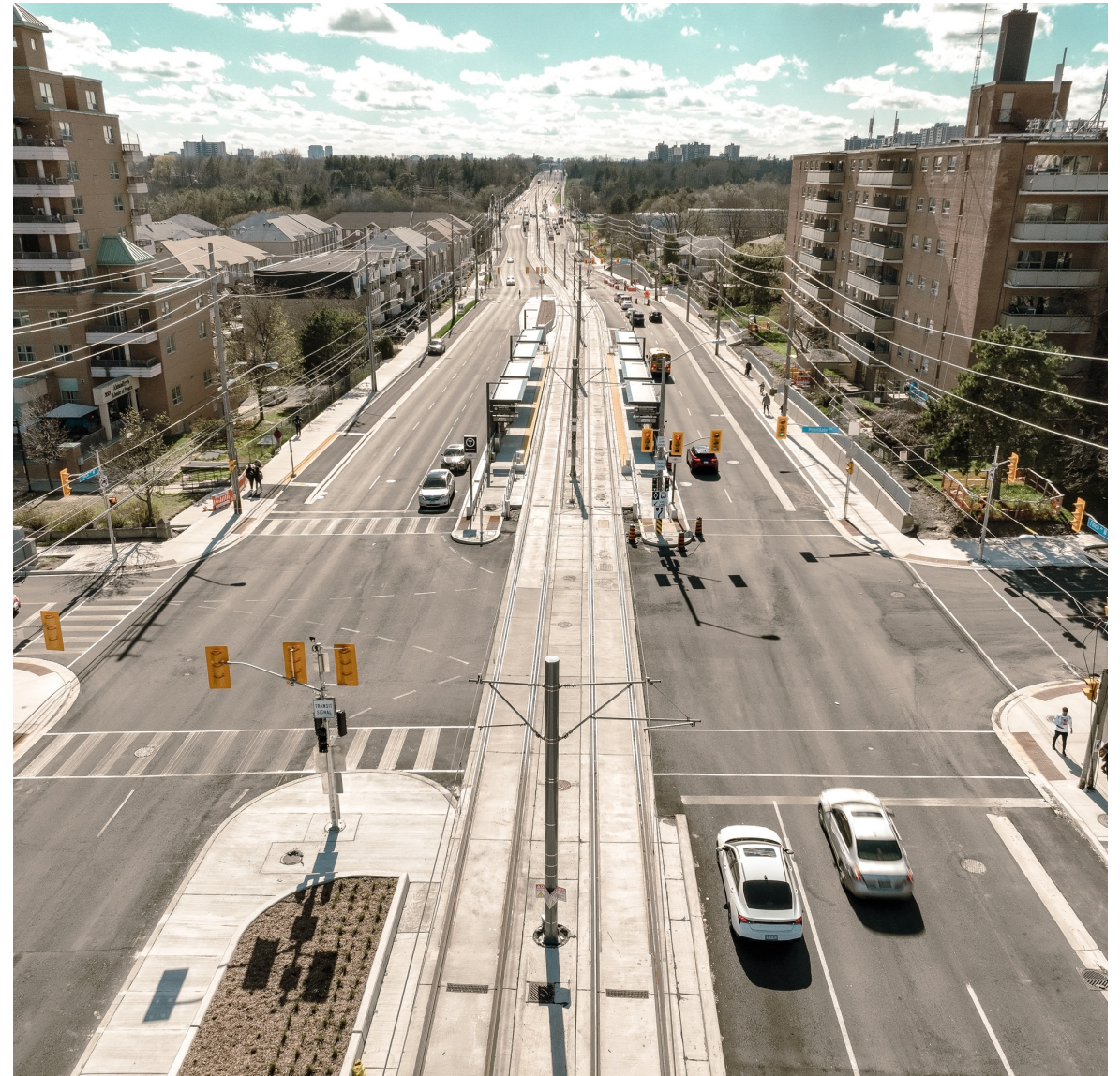
Photo: Finch Ave West and Pearldale Ave, aerial west view. 2024.04.27
