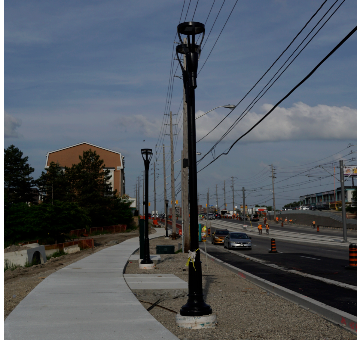
Photo: BIA Lamp posts newly installed at Lindy Lou Park. 2024.06.04
