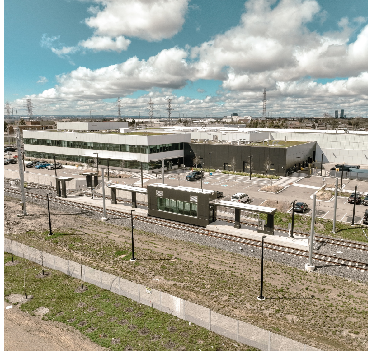
Photo: Maintenance and Storage Facility Handoff Platform northwest arial view. 2024.04.27
