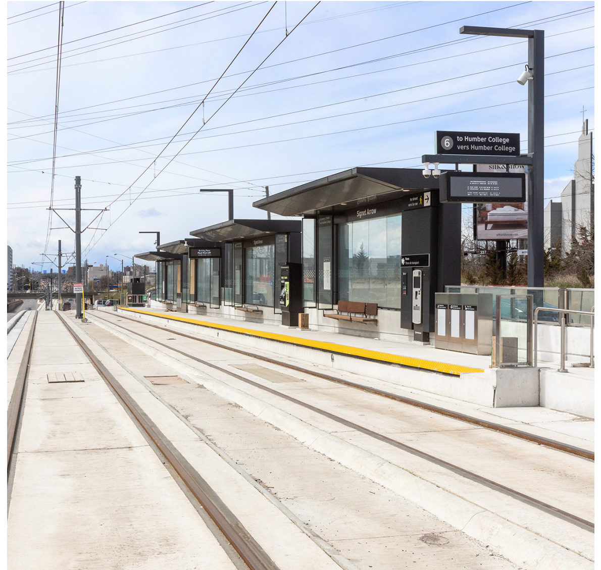
Photo: Signet Arrow stop westbound platform, west view 2024.04.27
