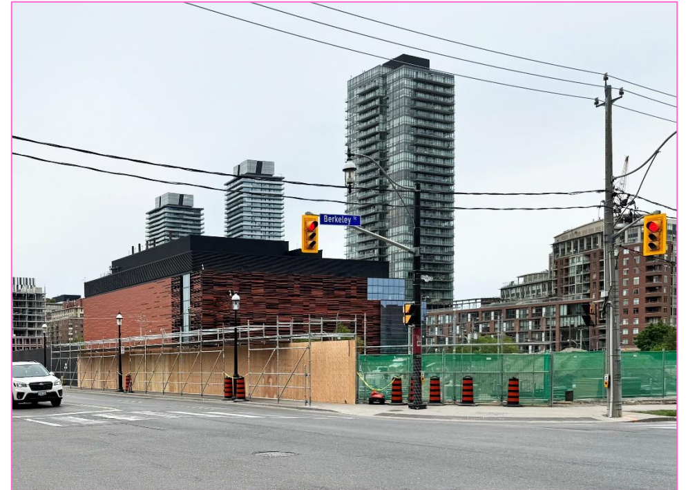
Pedestrian tunnel at Berkeley Street and Front Street East
