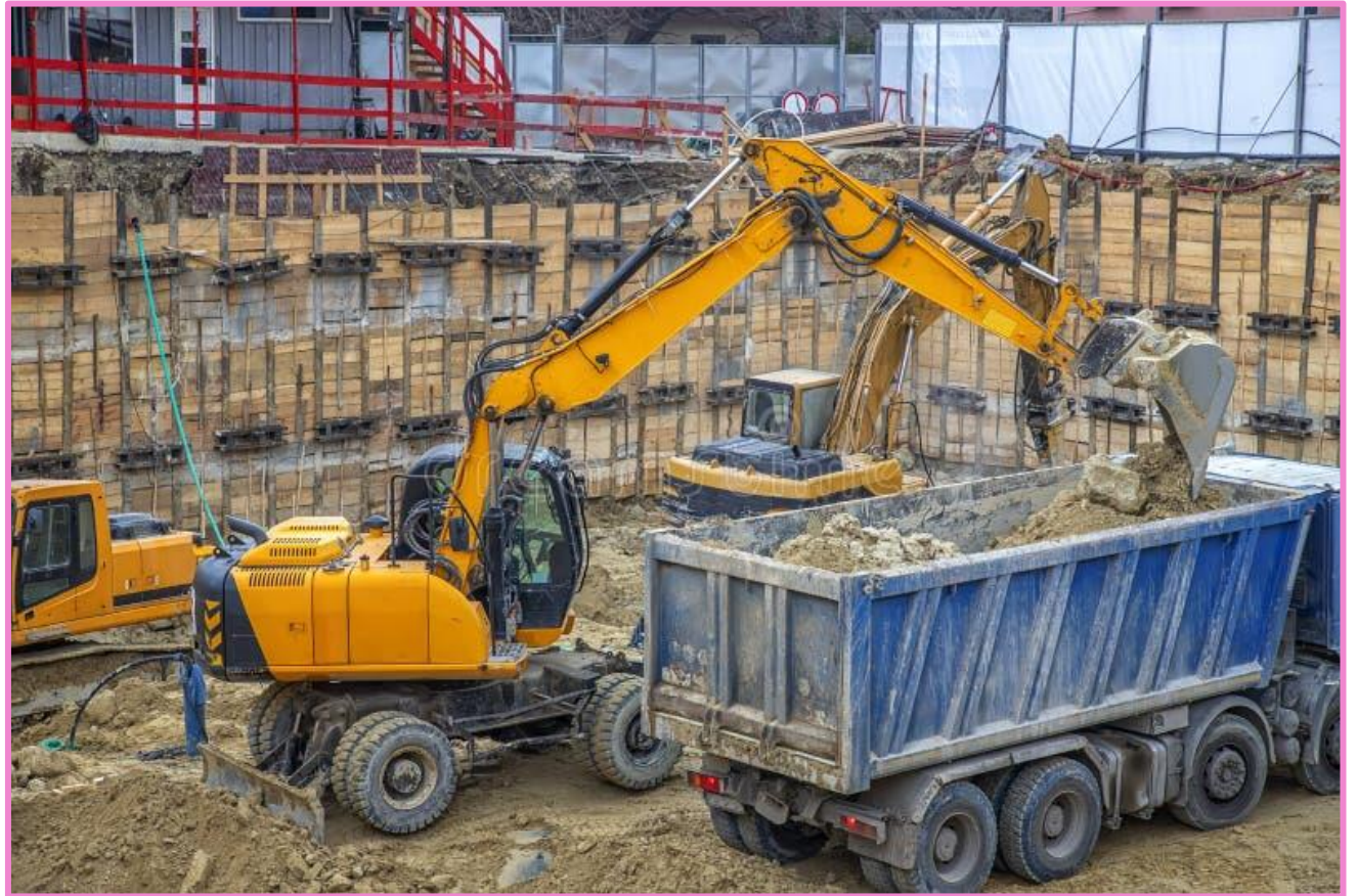
Excavated material being loaded into a dump truck.
