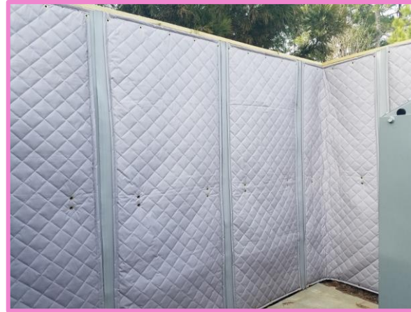
Sound dampening blankets place on the inside of site hoarding.
