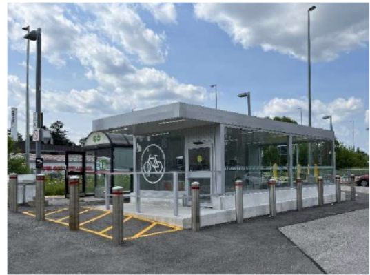
Enclosed bike room at Stouffville GO Station.
