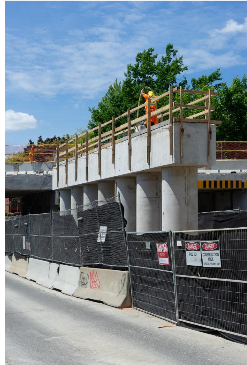
New piers at Dundas St. E.
