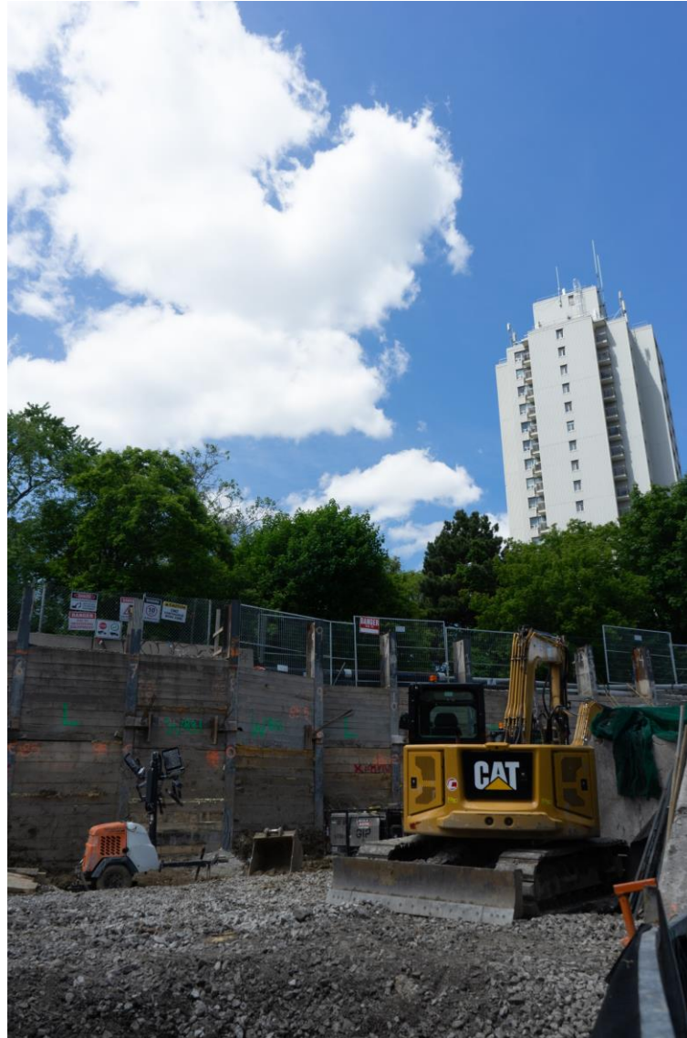
Progress on lagging.
