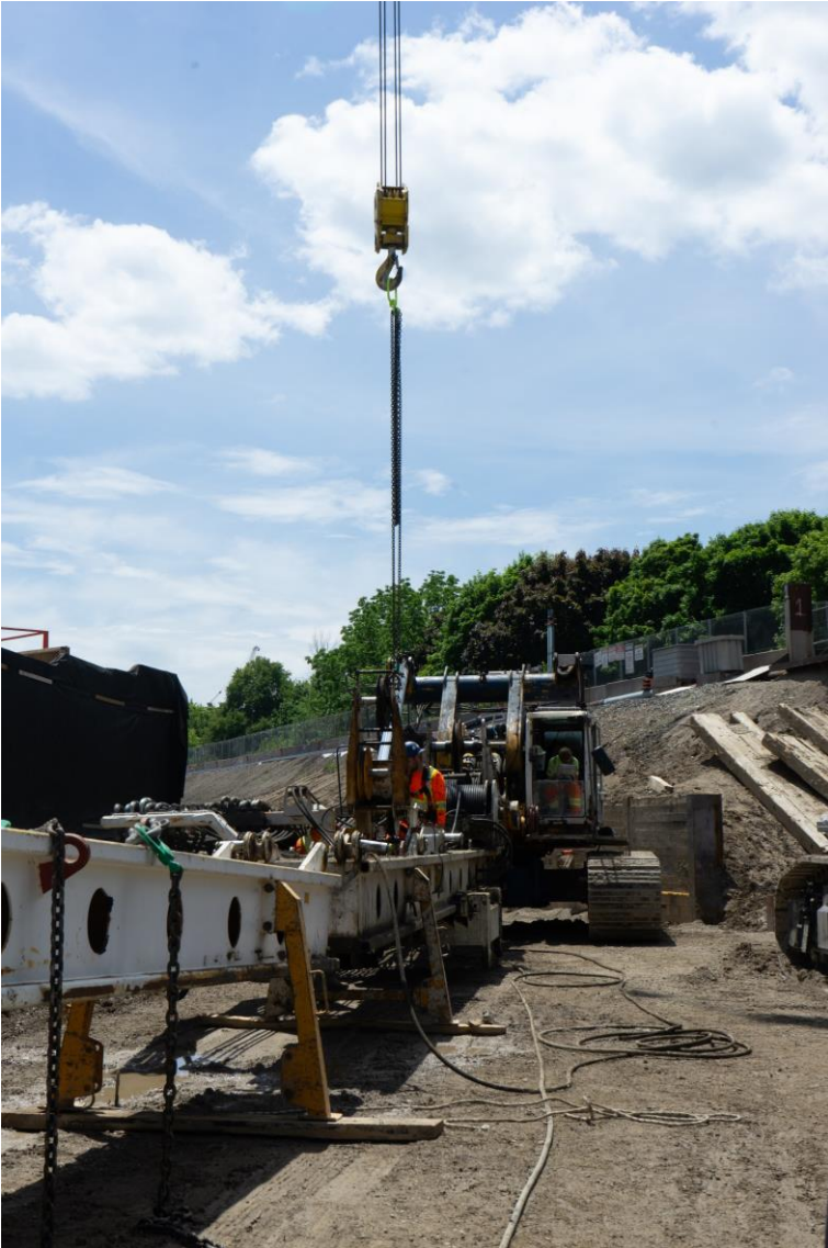
Setting up a crane for new abutments
