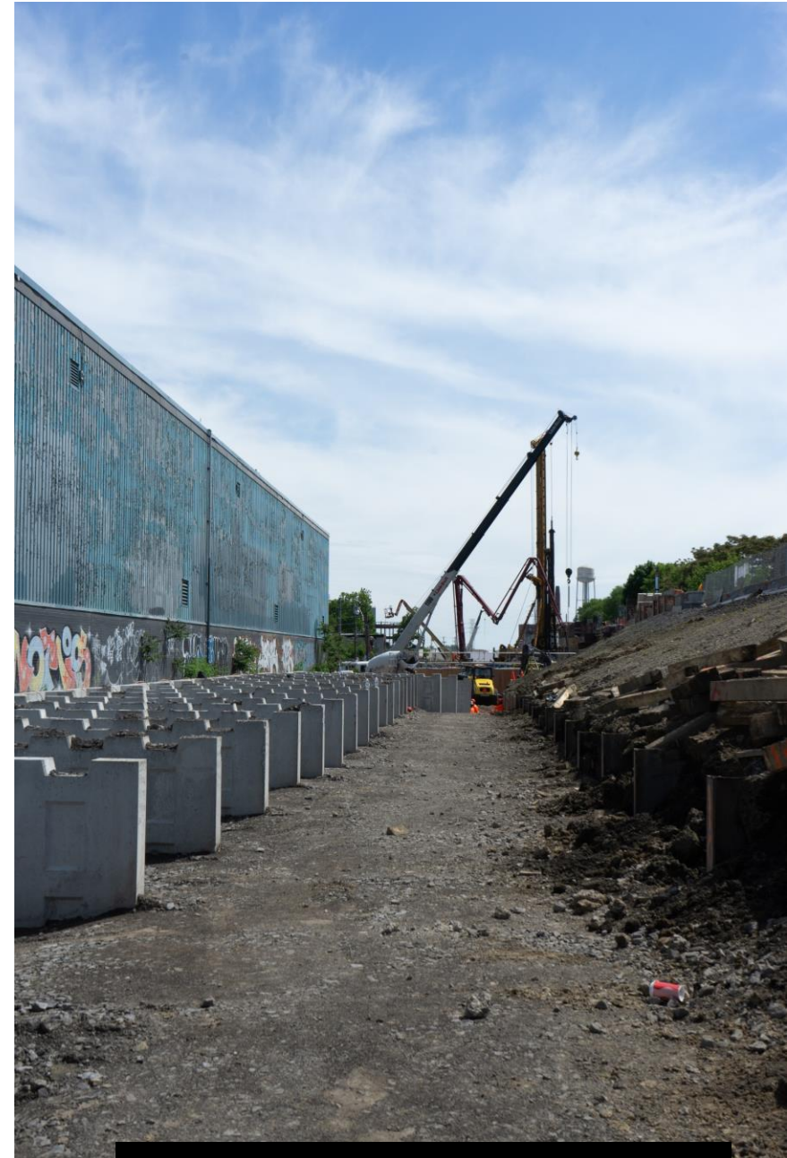
May 29, 2024 Retaining wall and bridge work
