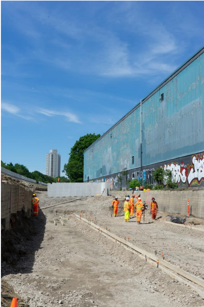
Preparing the next set of blocks
