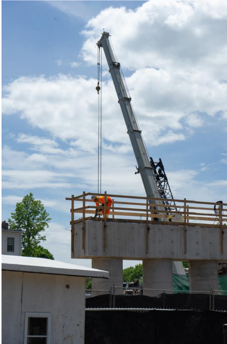
Putting in the final touches on the new piers
