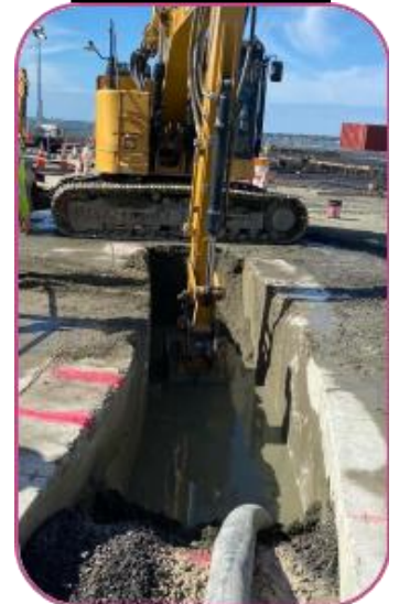
Excavation with slurry
