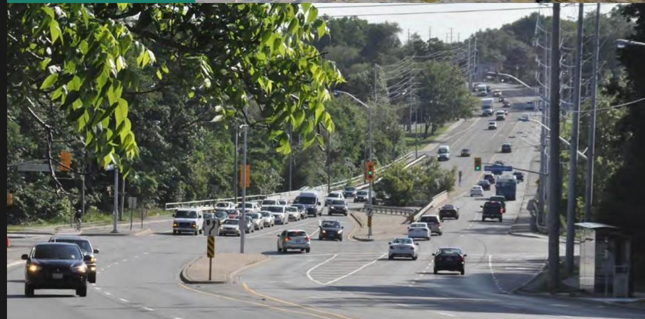
Erindale Valley and Credit River Bridges
