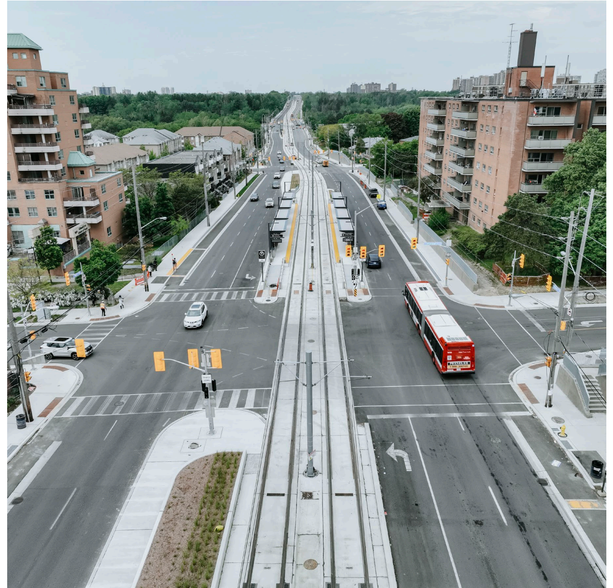
Photo: Finch Ave West and Pearldale Ave, aerial west view. 2024.05.21
