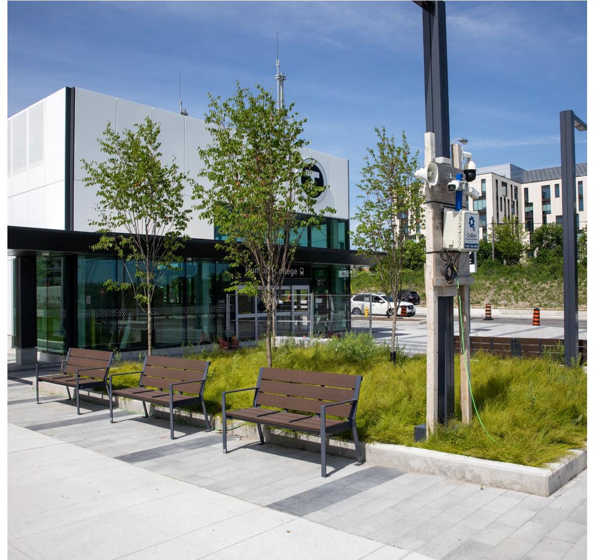
Photo: Humber College station south building exterior. 2024.05.21
