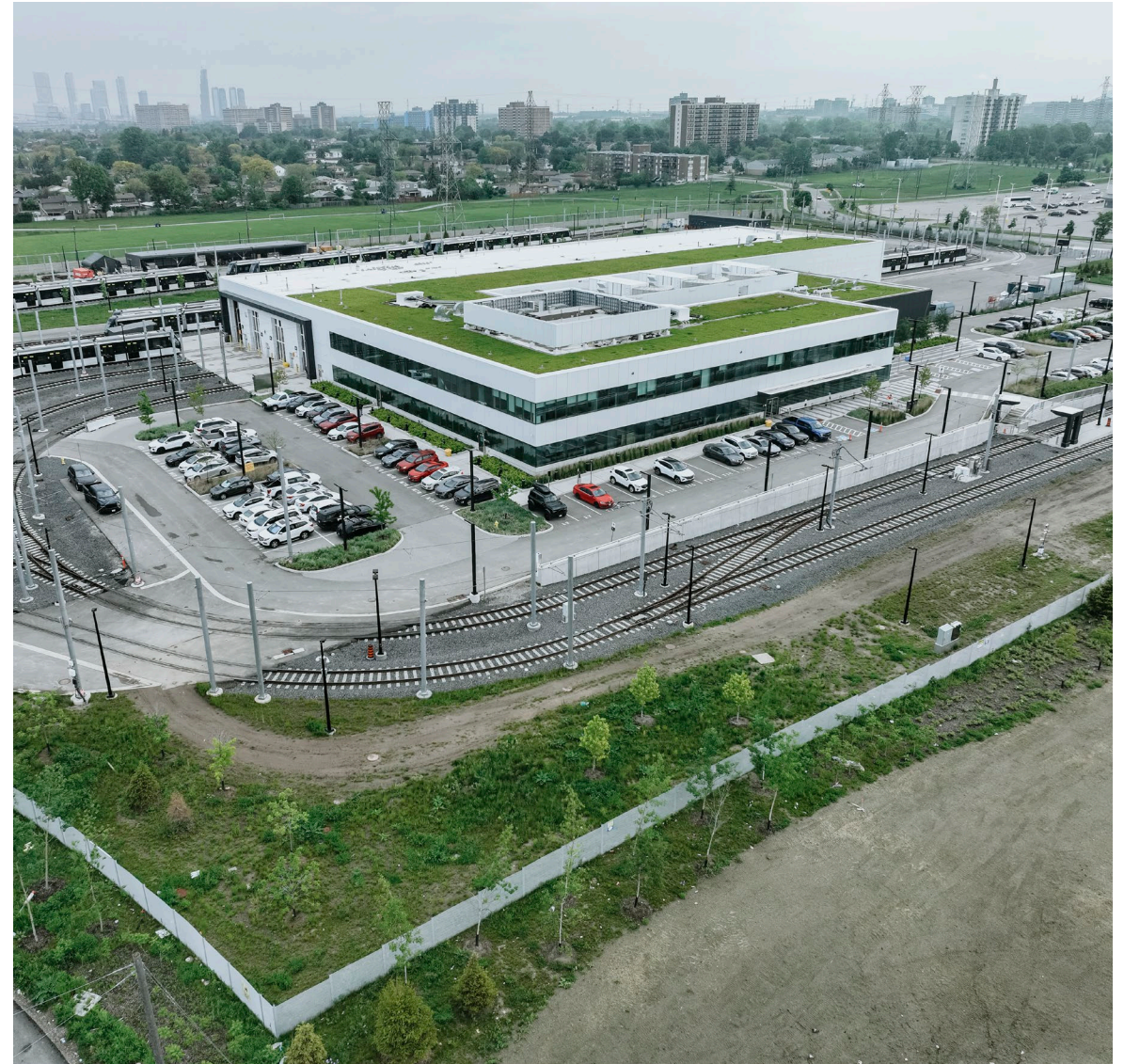
Photo: Maintenance and Storage Facility , northeast arial view. 2024.05.21
