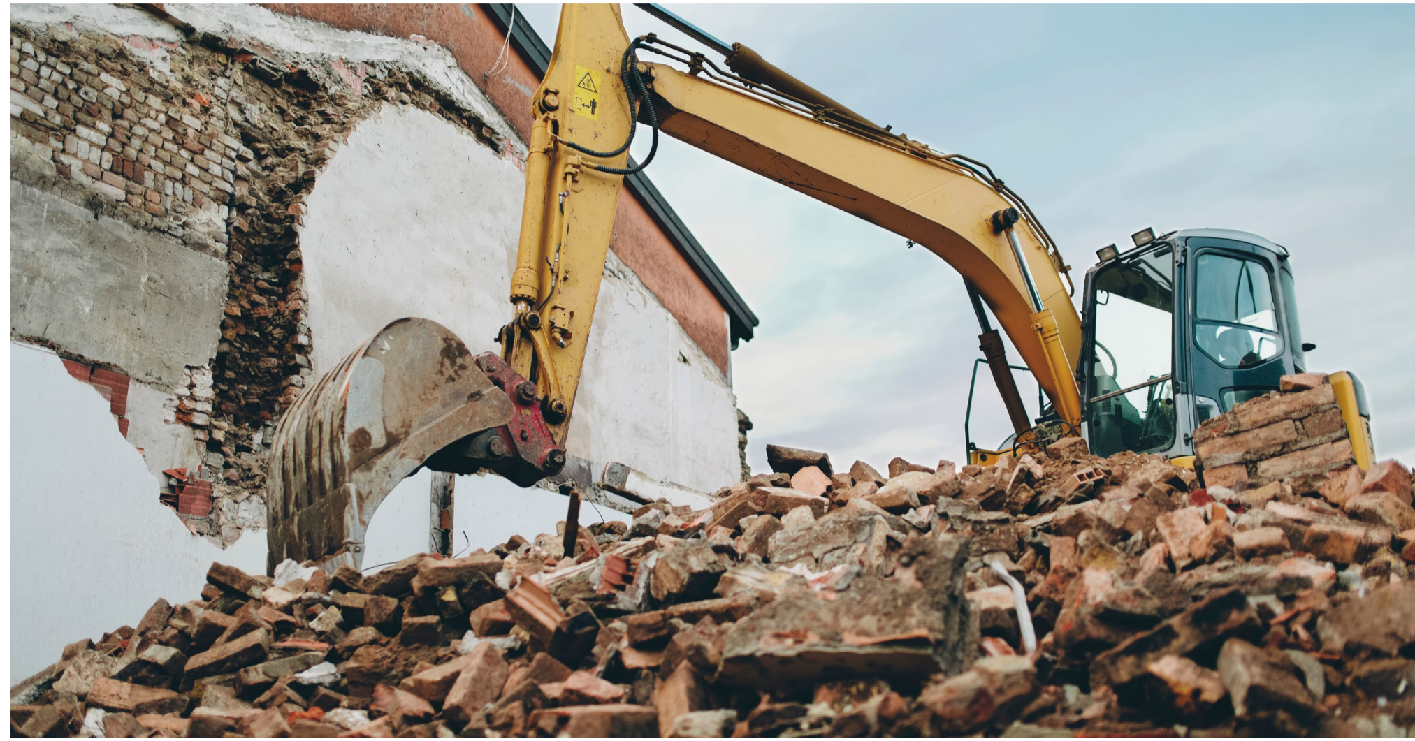
1 Demolition (449 Carlaw plaza and 388-402 Pape Ave)
