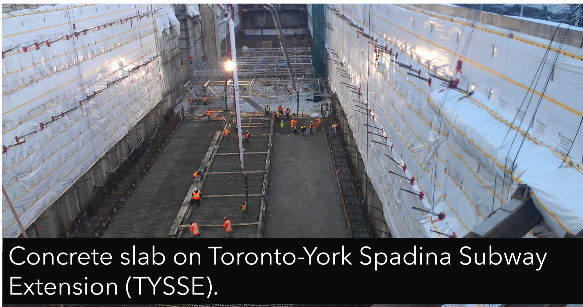
4 Excavation of the portal footprint and installation of a concrete slab to act as a cradle for the TBM
