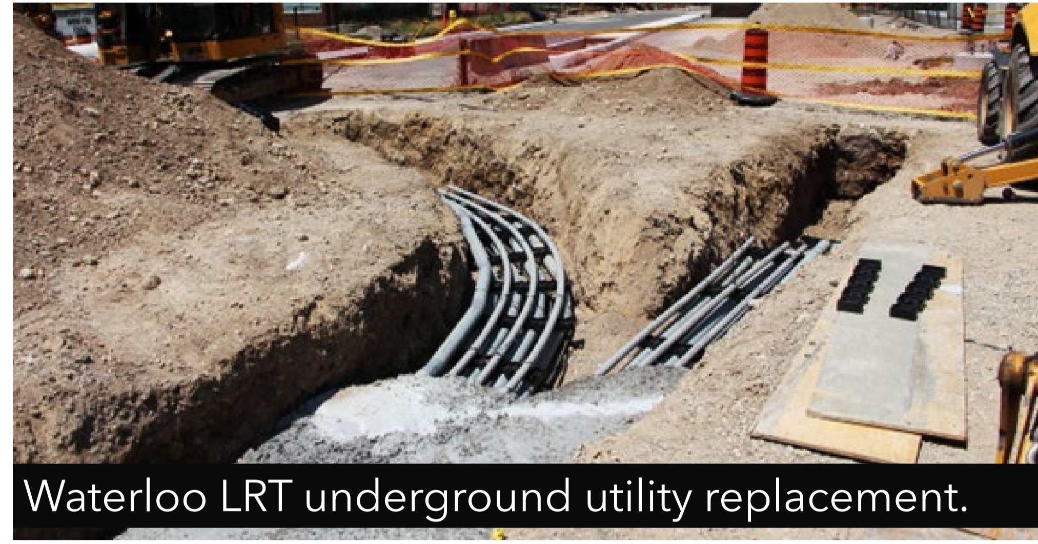
2 Underground utilities relocated (hydro, Rogers/ Bell, water, storm and sanitary sewer)
