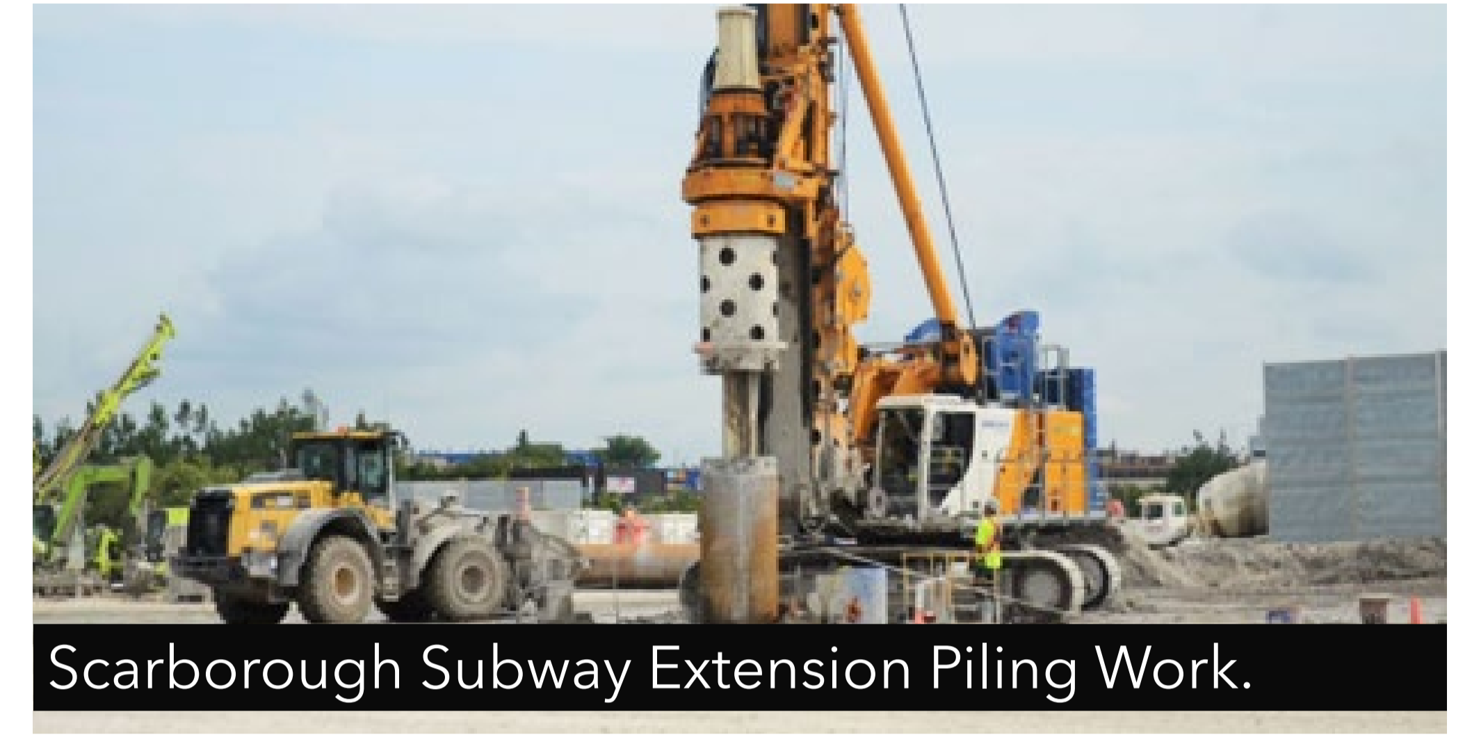
3 Drilling piles to support excavation
