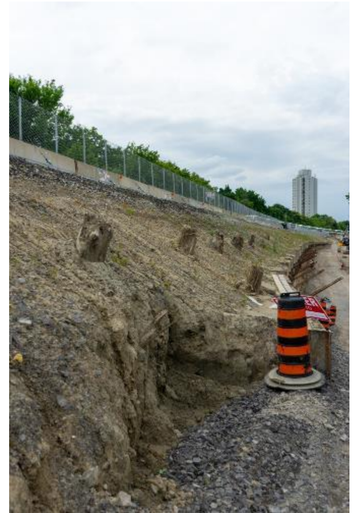
Original wooden piles emerging
