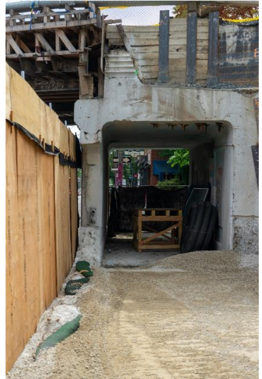
Queen St. E. with demolished abutment.
