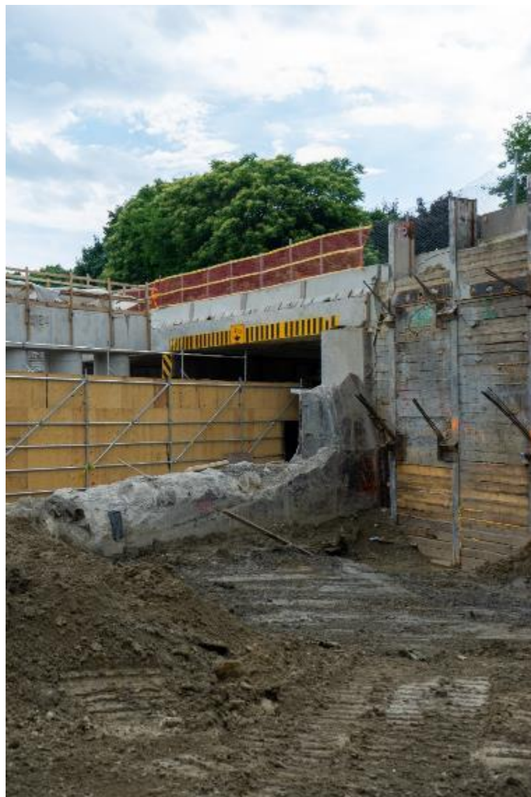
Abutment on north side of Dundas St. E. (now demolished)
