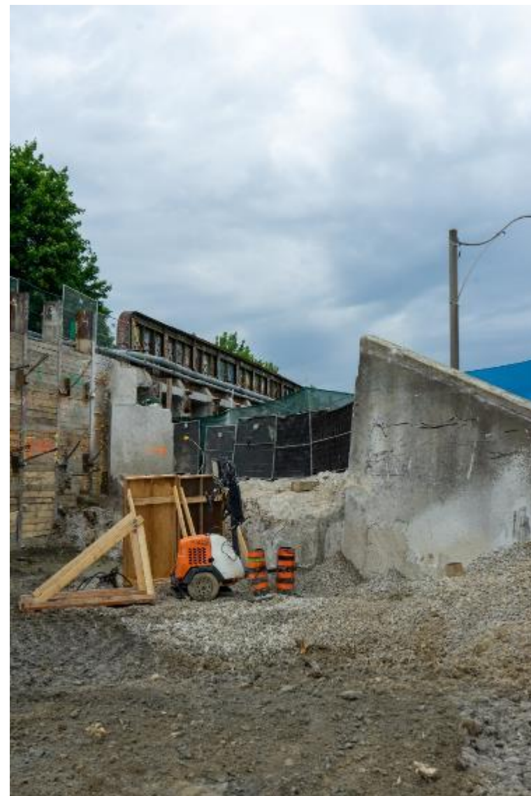
Abutment on west side of Logan Ave.
