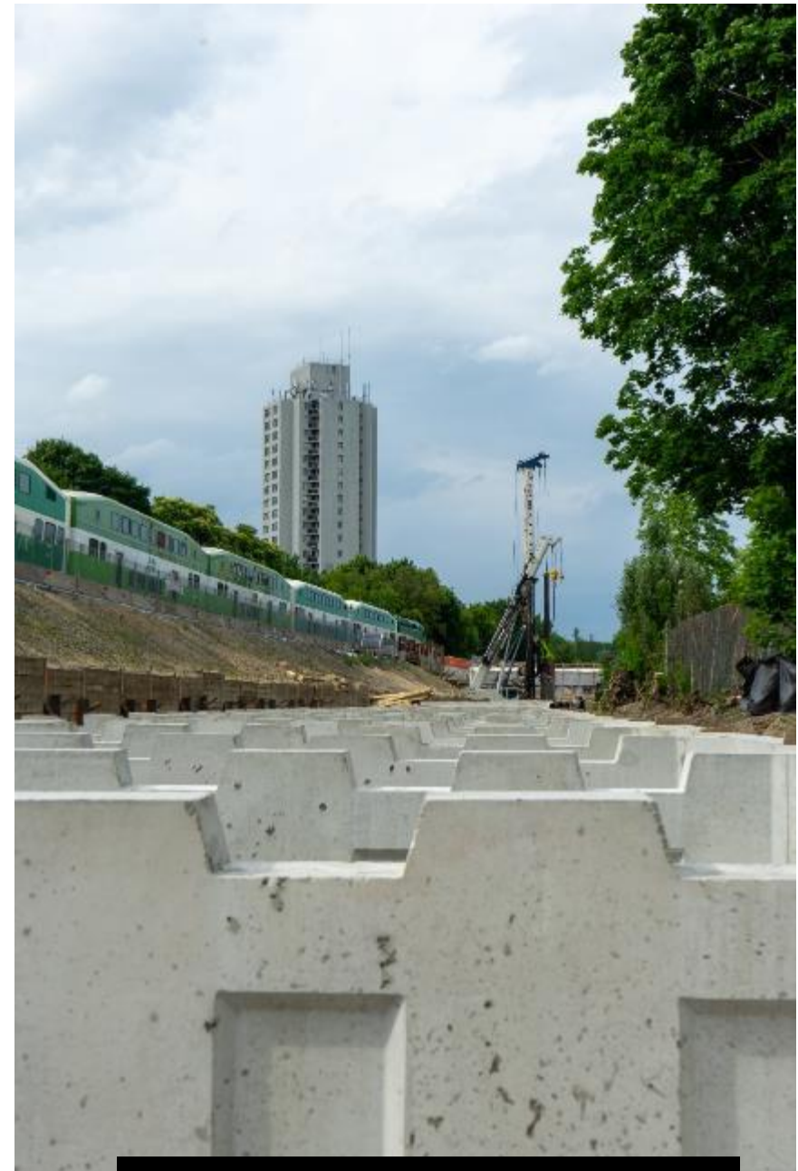
June 25, 2024 Retaining wall work
