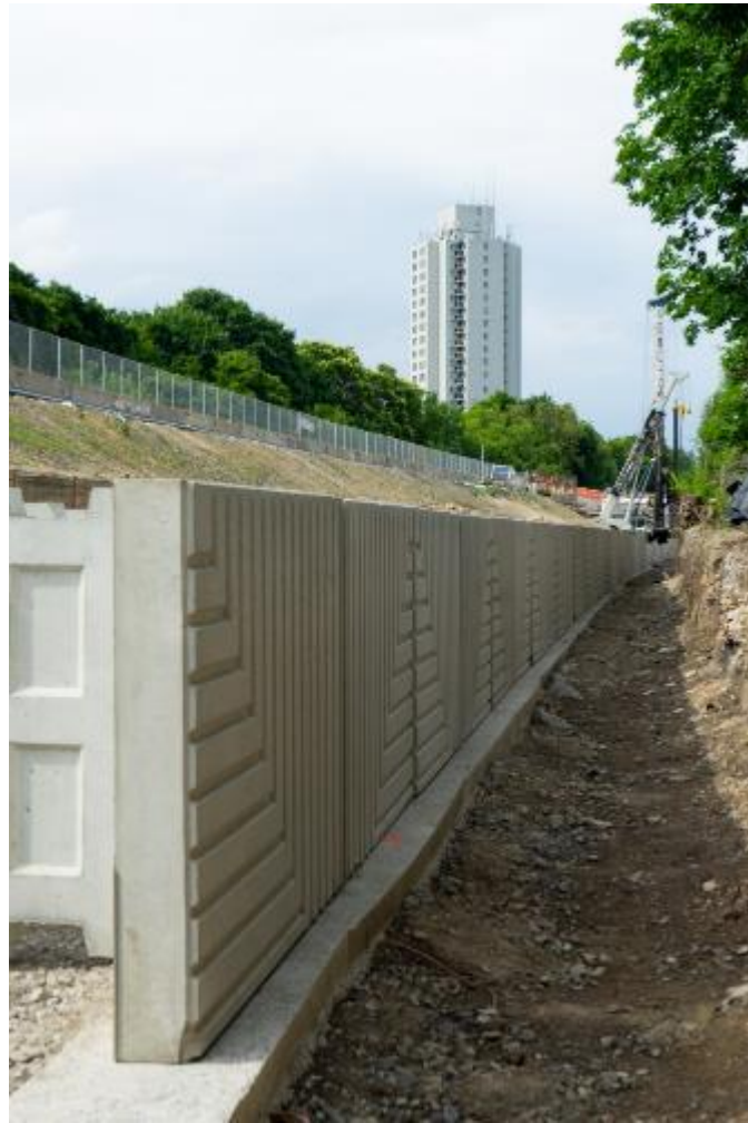
First row of retaining walls with precast pattern
