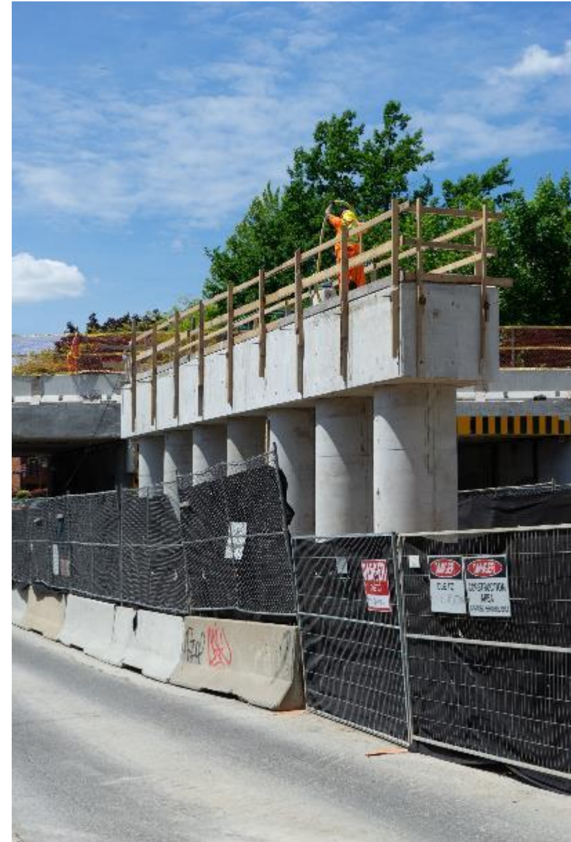
New piers at Dundas St. E.
