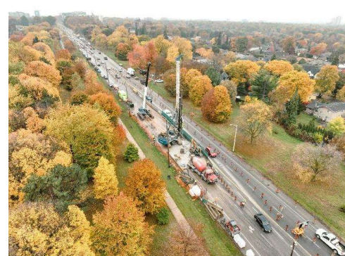
Additional Headwall (Russell Rd)
