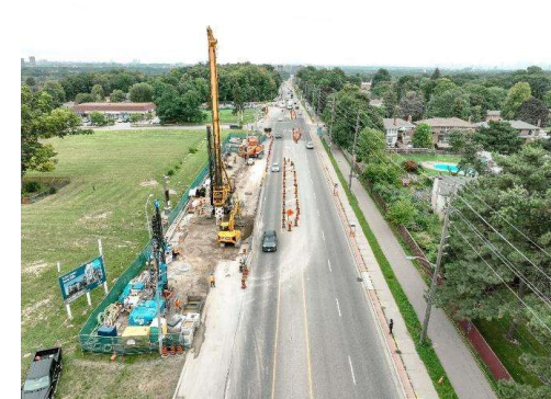
Additional Headwall (Wincott Dr)
