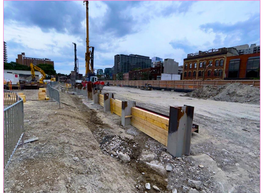
Timber lagging installation in the structural beams
