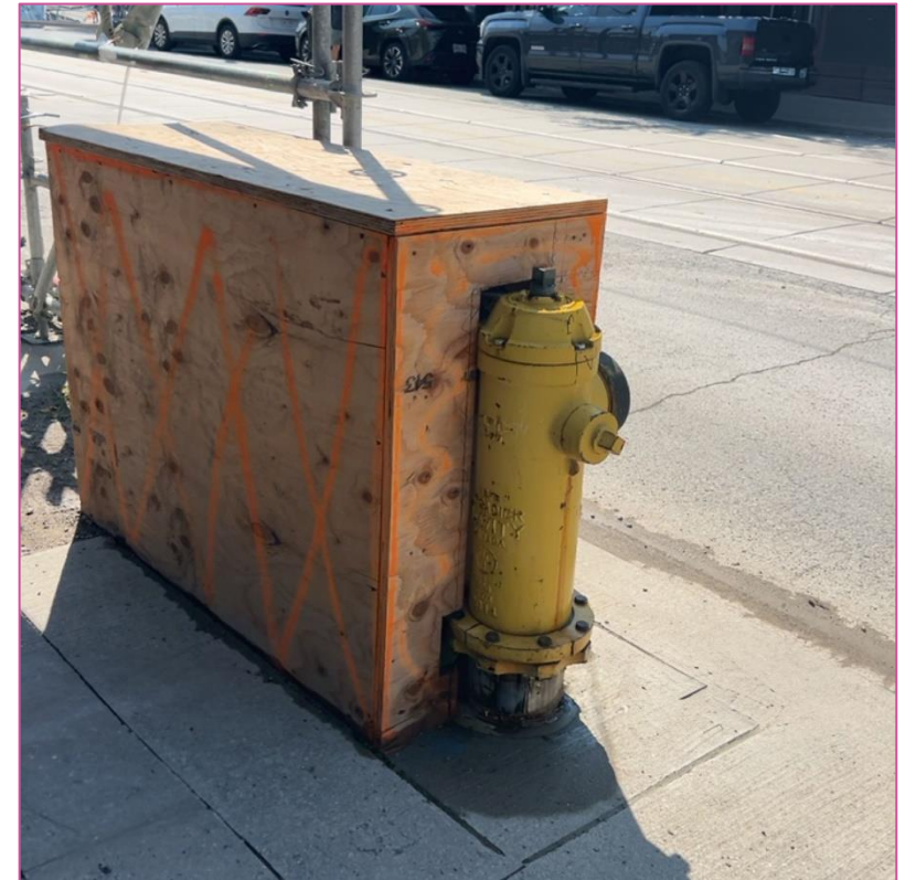
Protecting the fire hydrant connection
