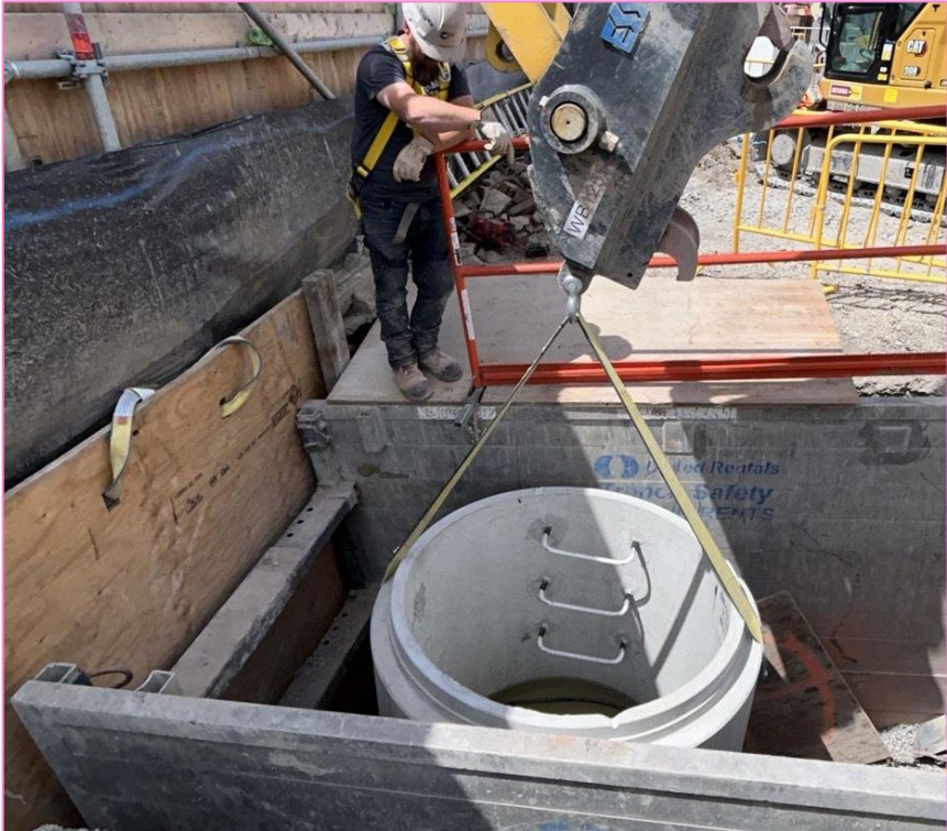
Manhole installation for water management within the site.
