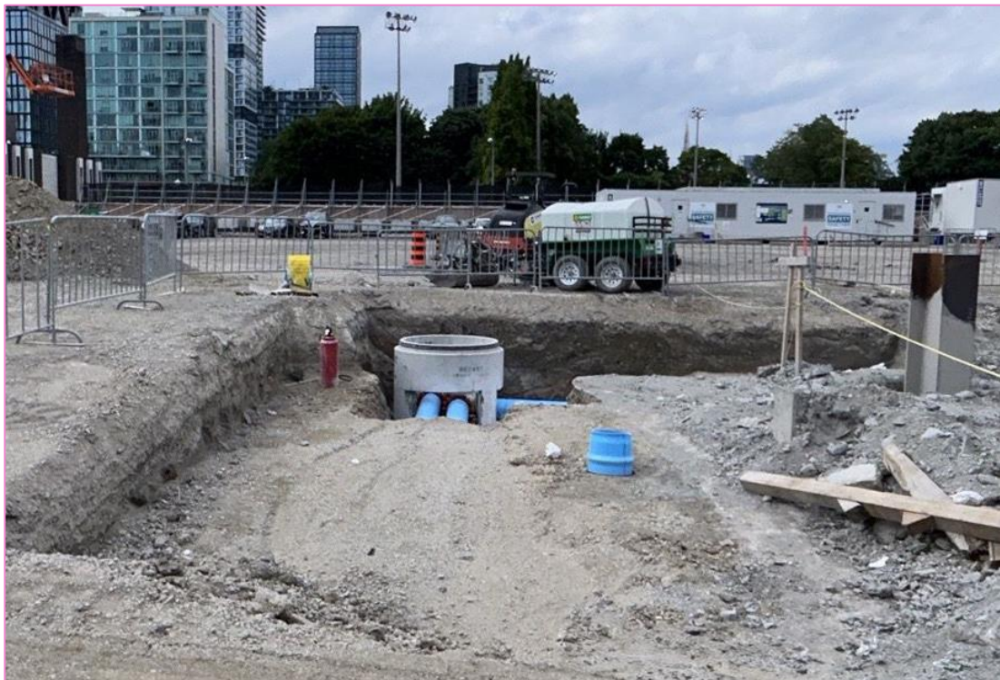
Water by-pass installation around the shaft.
