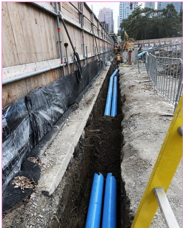
Pipe installation parallel to shaft and hoarding.
