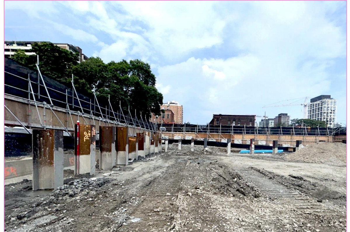
Structural beams along the shaft perimeter
