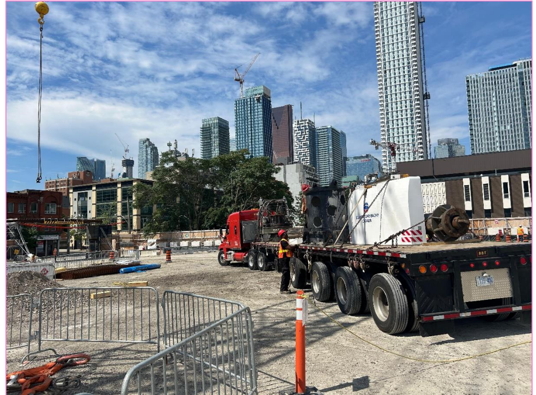
Drill rig 1 demobilized and ready for relocation
