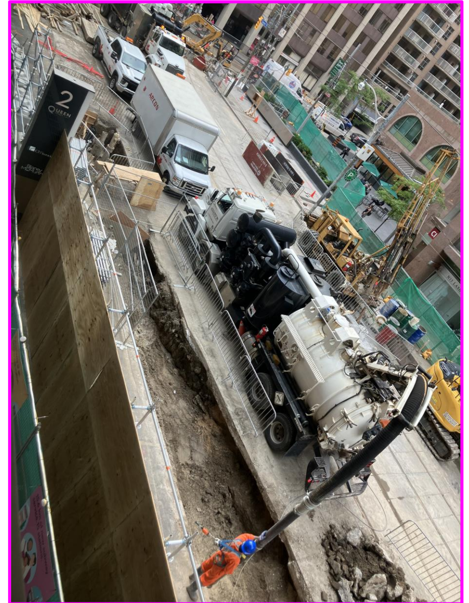
Example of a sewer investigation in progress in the East.
