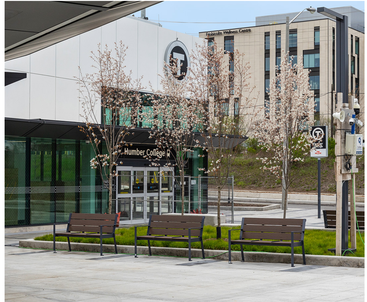
Photo: Humber College station exterior south building. 2024.04.27
