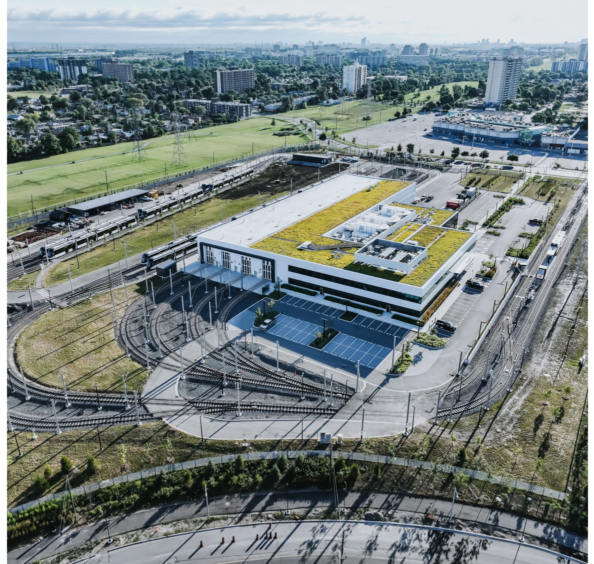
Photo: Maintenance and Storage Facility, northeast aerial view. 2024.06.22
