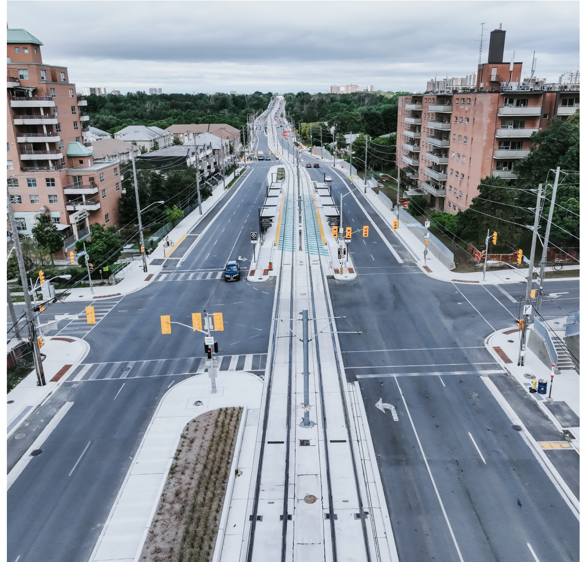
Photo: Finch Avenue West and Pearldale Avenue, aerial view west. 2024.06.22
