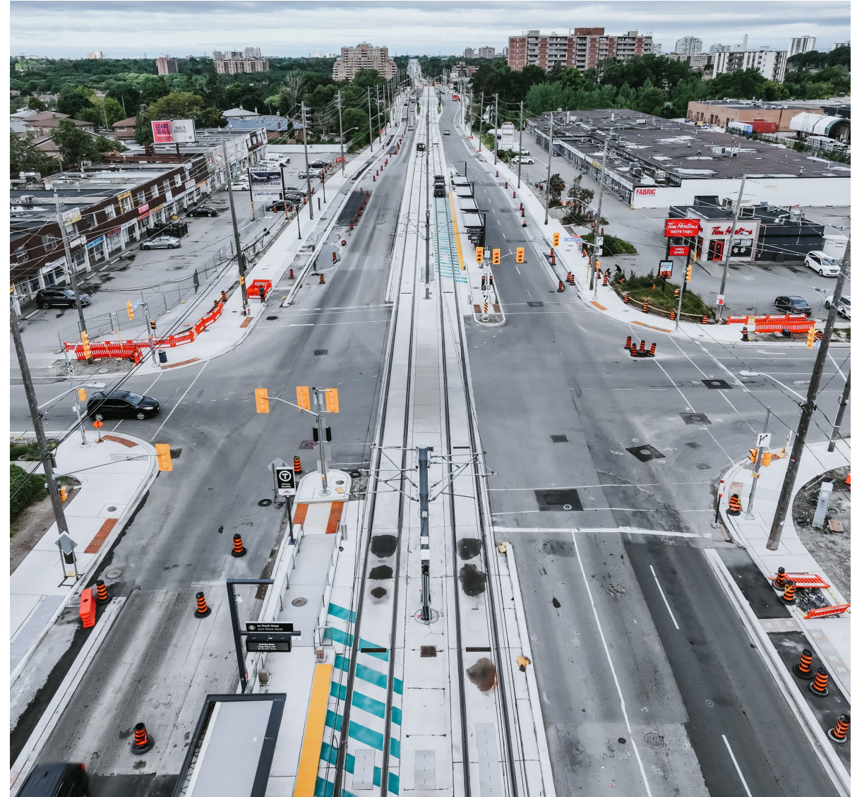
Photo: Finch Avenue West and Milvan Drive, aerial view west. 2024.06.22
