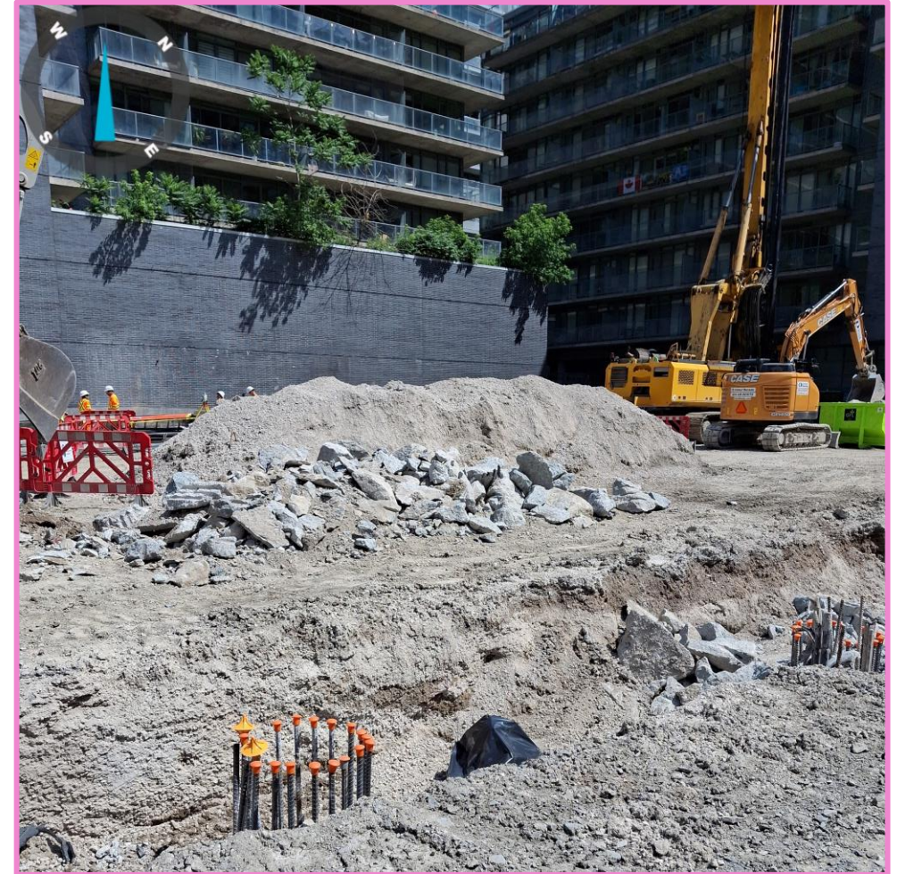
Pile drilling machine and excavator at King-Bathurst.
