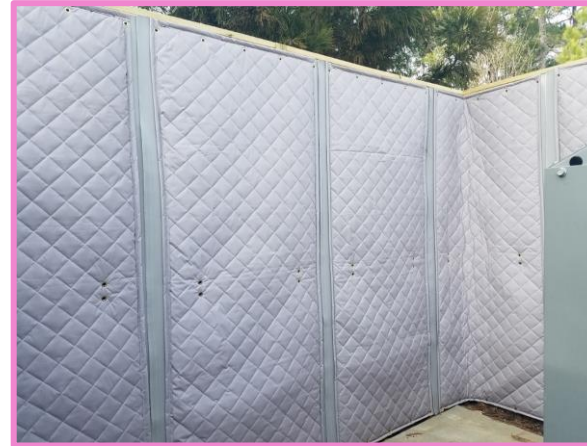
Sound dampening blankets placed on the inside of site hoarding.
