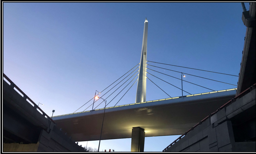
St-Jacques Bridge (Montreal, Québec) - Completed 2018
