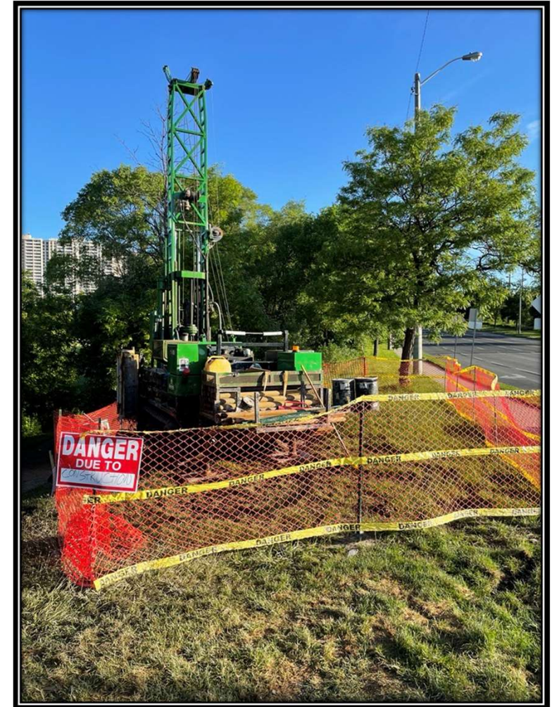
Borehole drilling along the elevated guideway
