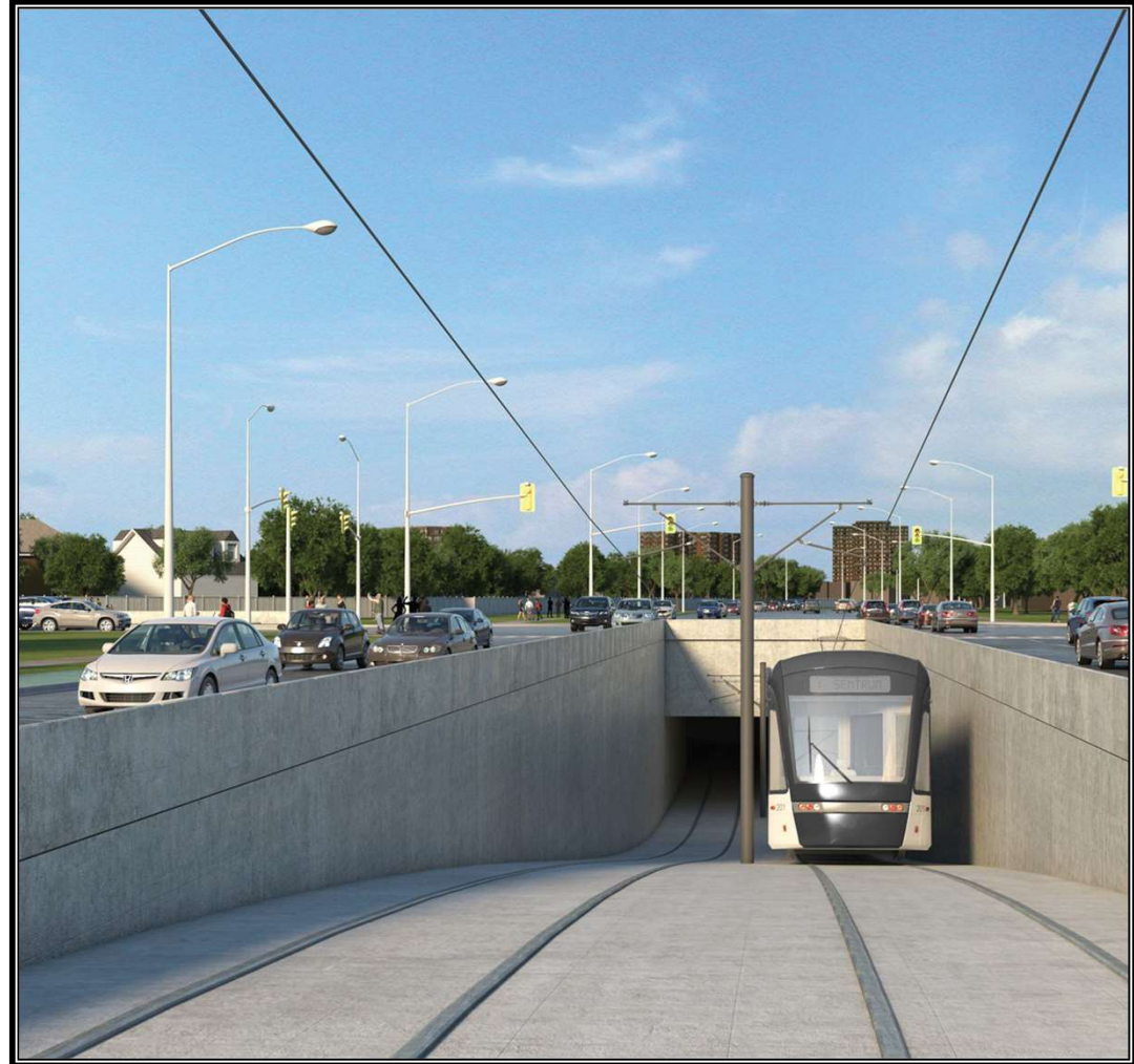
Humber College portal at Finch West LRT project, Toronto
