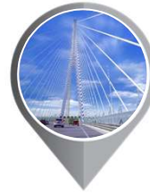
2018* GORDIE HOWE INTERNATIONAL BRIDGE
