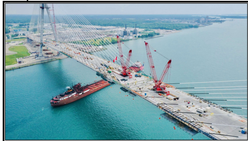
Gordie Howe International Bridge (Detroit, Michigan/Windsor, Ontario) - Under Construction
