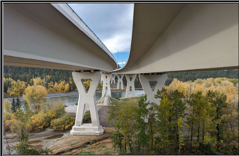
Bow River Bridge Twinning Project (Calgary, Alberta) - Completed 2023
