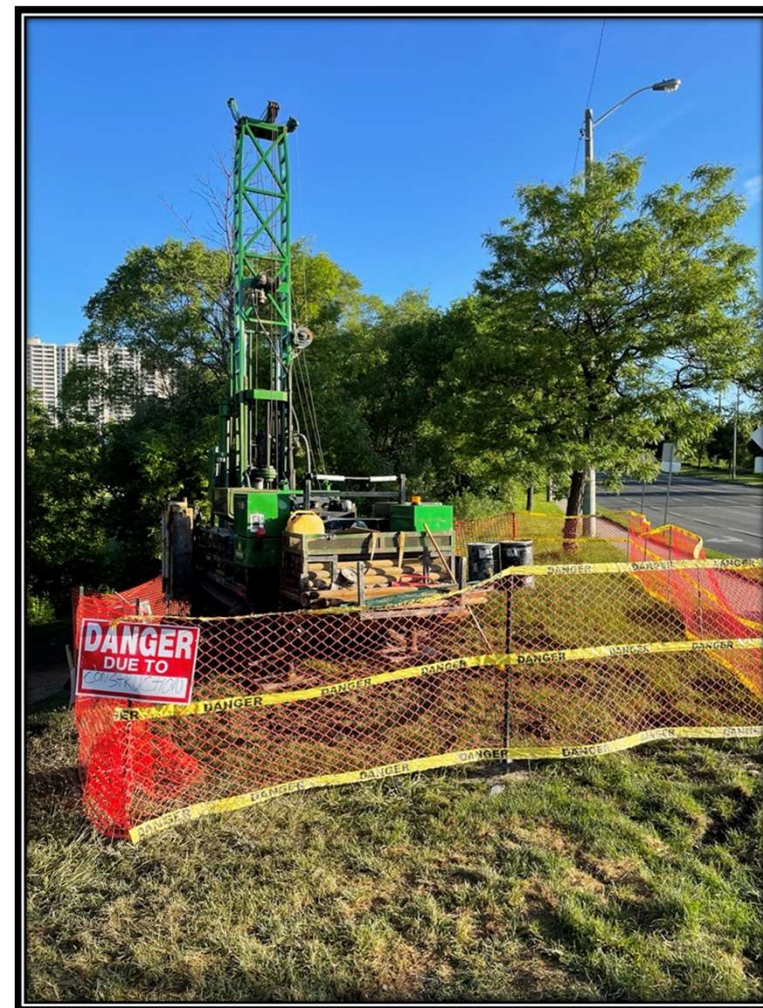
Borehole drilling along the elevated guideway
