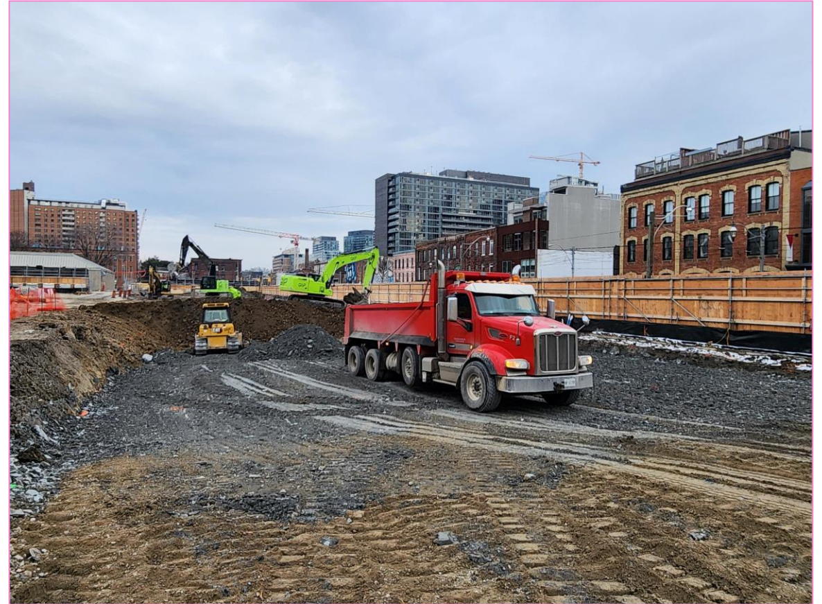
Excavation of the working platform in the initial stages
