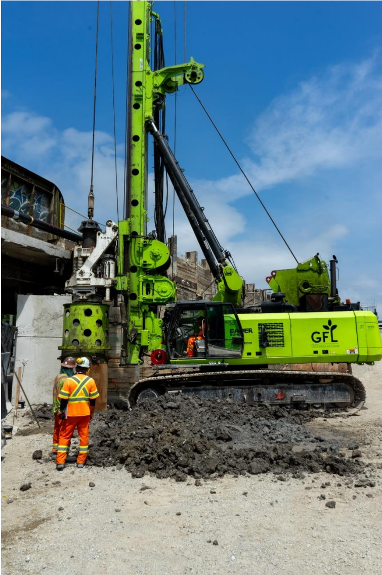
Caisson drilling on the east abutment at the Logan bridge
