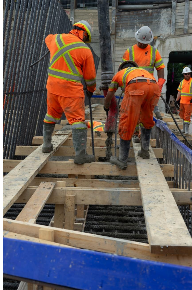
Concrete vibrators are inserted during the pour to remove air bubbles
