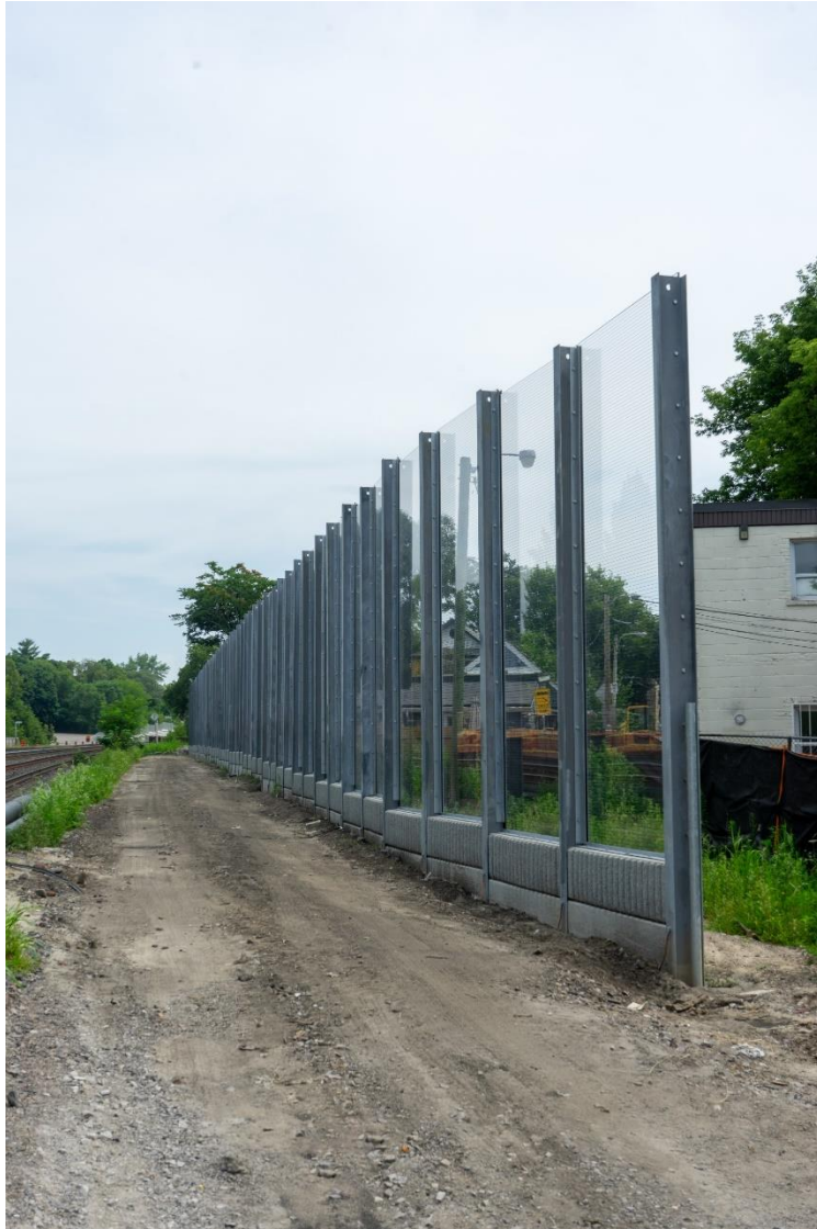
Completed noise barrier installed at Galt Ave.
