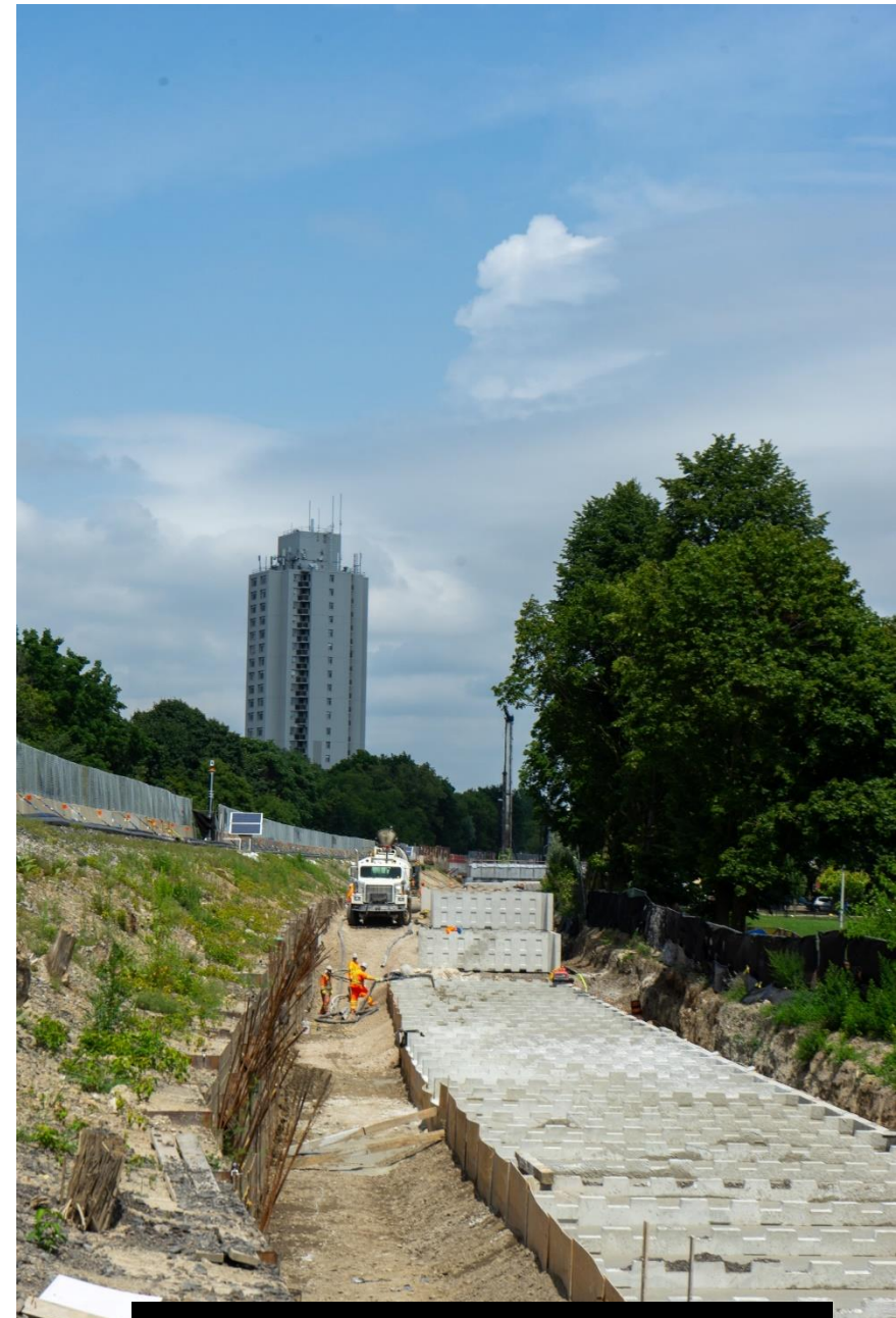
July 30, 2024 Retaining wall work
