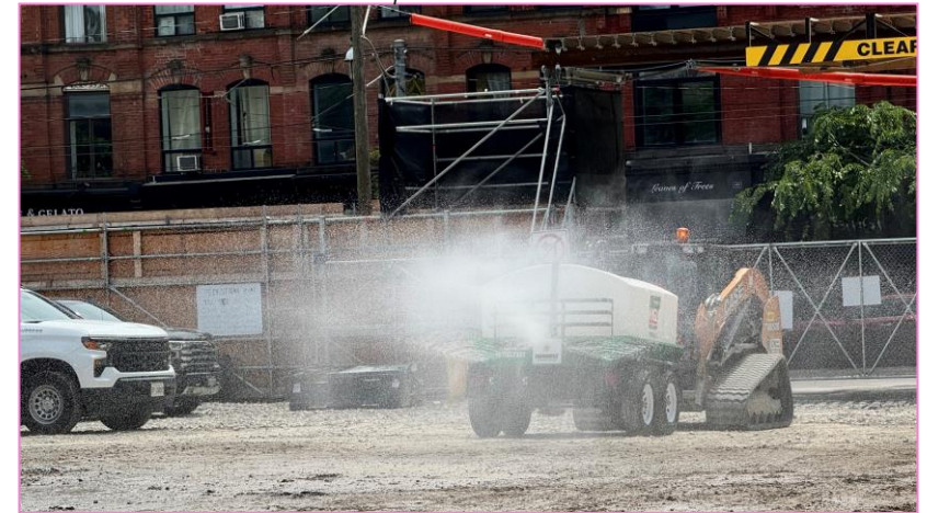
Example of dampening soils to suppress dust
