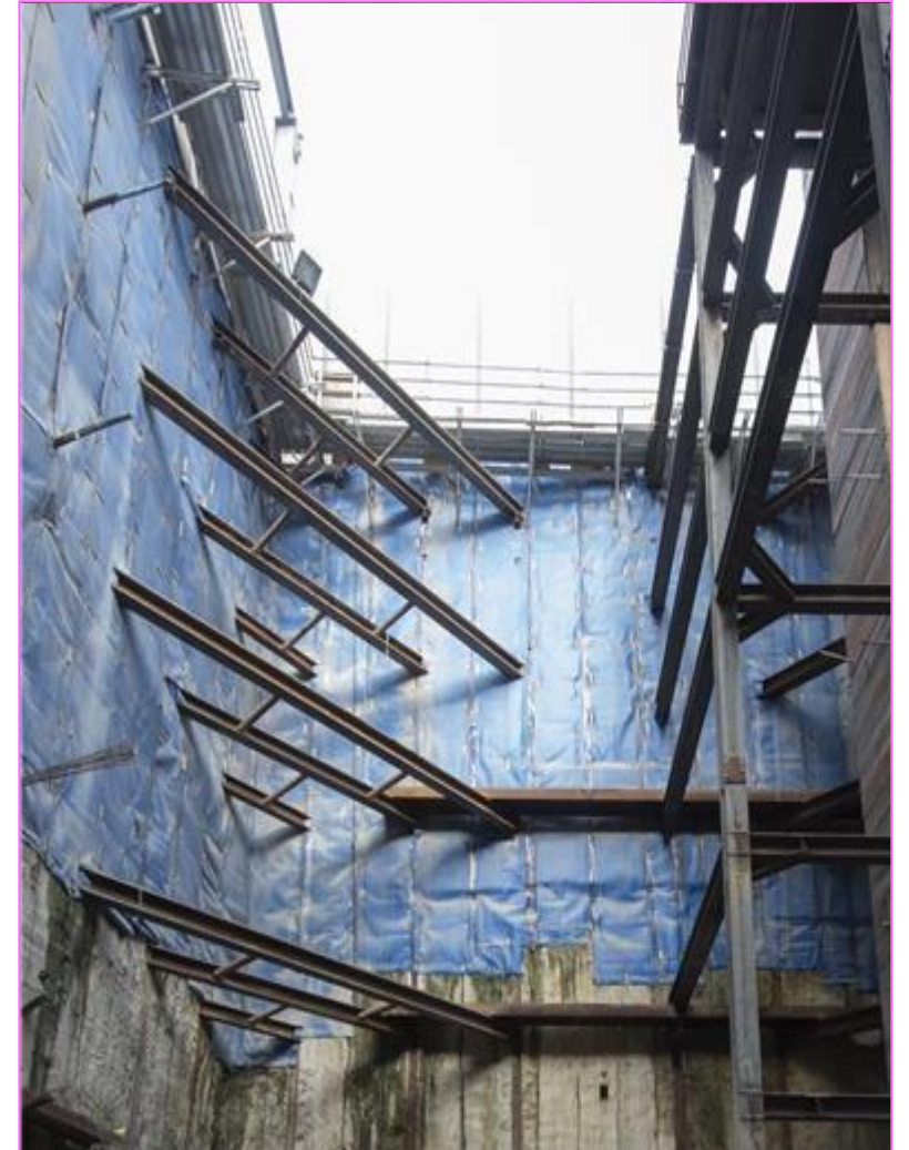
Example of shaft excavation, with walers and struts.
