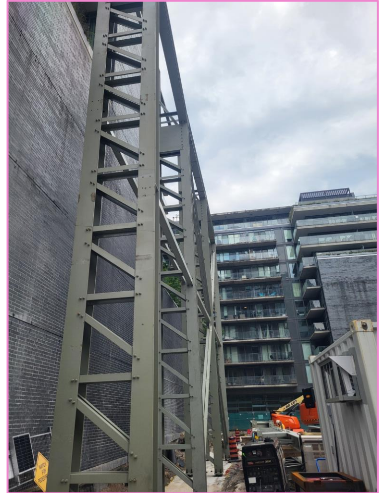
Example of an acoustic shelter installation in progress
