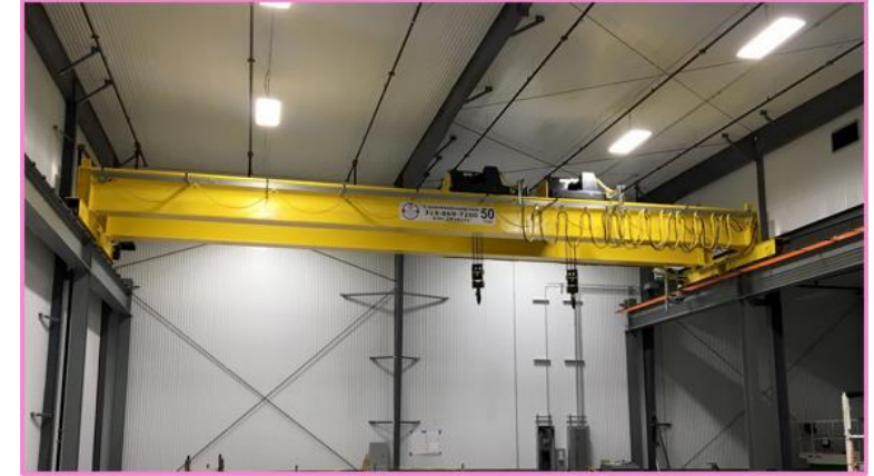
Example of an overhead crane used inside of an acoustic shelter during excavation
