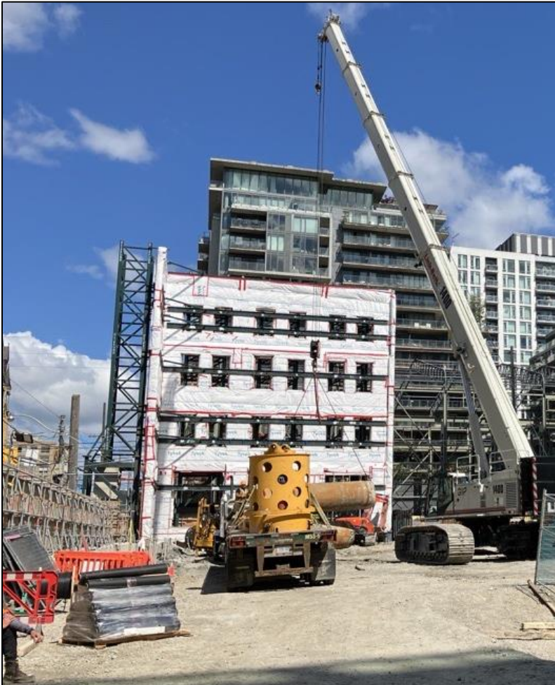
Drill rig disassembly and removal in process from King-Bathurst.
