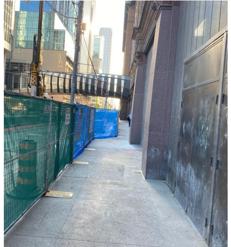
Hydro vault street-level work completed on July 26, 2024
