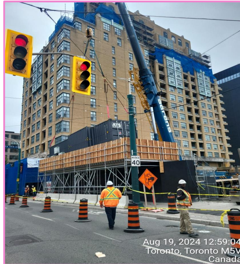
Installation of the power substation on the overhead platform
