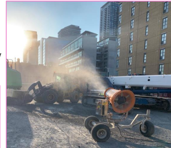
Water spray machine to reduce dust
