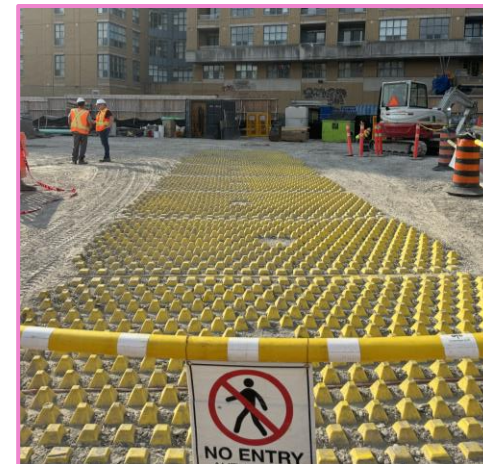
Mud mat in place to reduce dust
