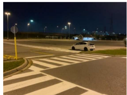
New pedestrian crossing pavement markings at Langstaff GO Station.
