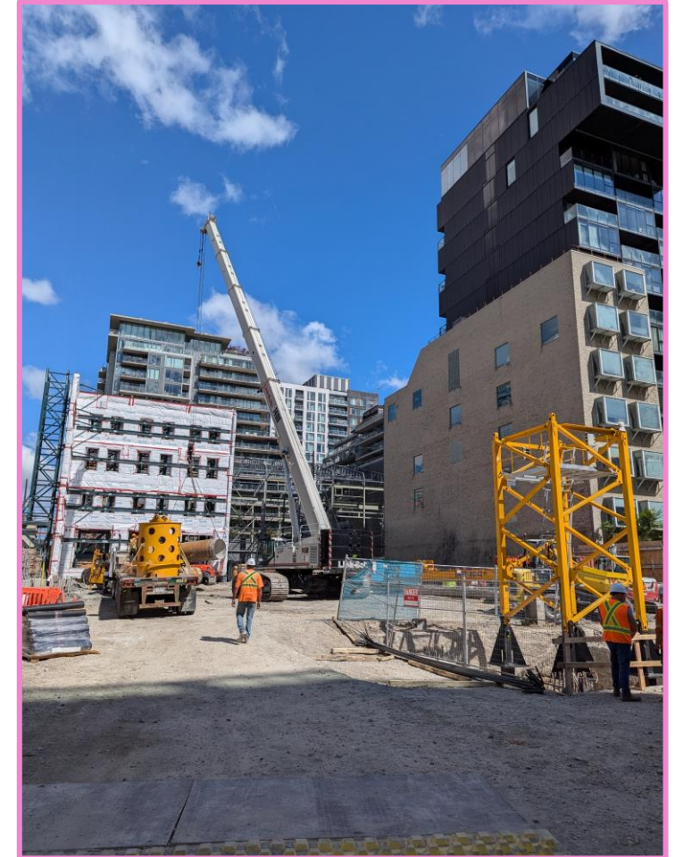
Pile drilling machine being disassembled and removed from King-Bathurst (south).
