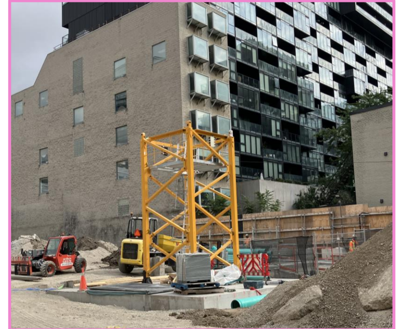
Tower crane base being installed at King-Bathurst (south).
