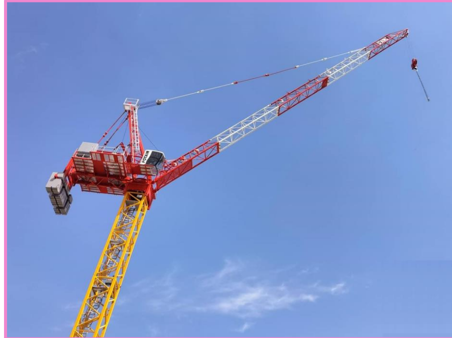
Example of a completed tower crane.
