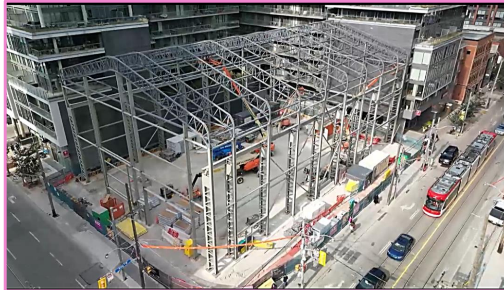
Assembly of the acoustic shelter structure.
