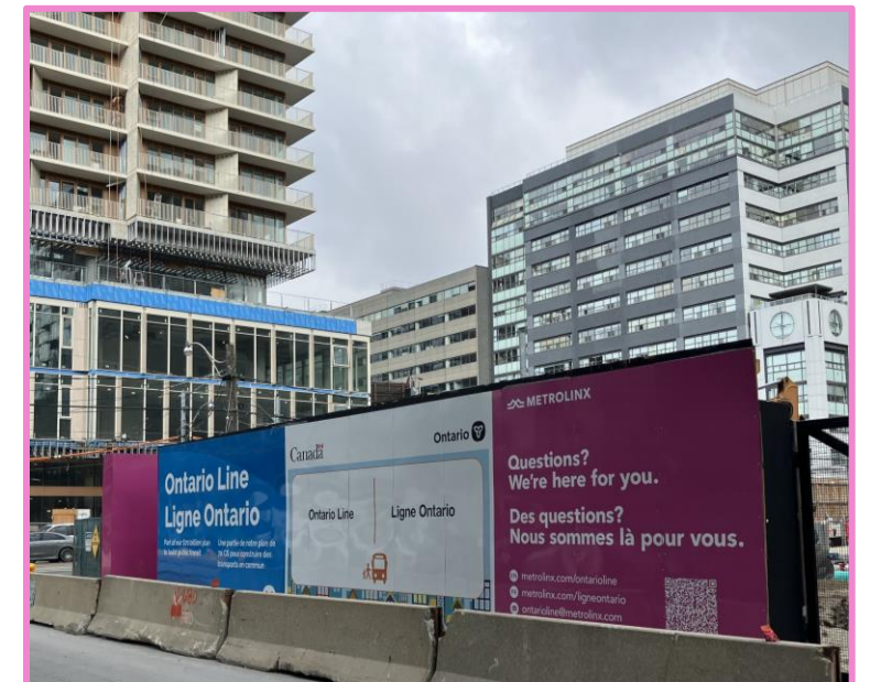
Hoarding installation at the south site.
