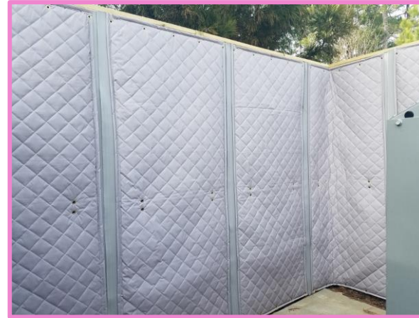
Sound dampening blankets to be placed on the inside of site hoarding.
