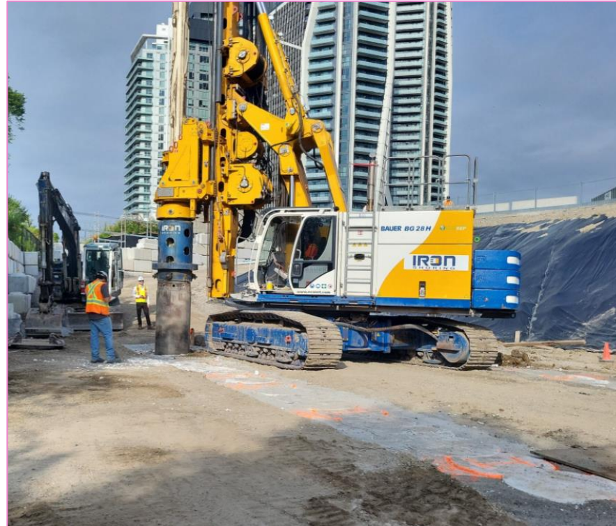
Left: Piling works underway at Ordnance Park.
