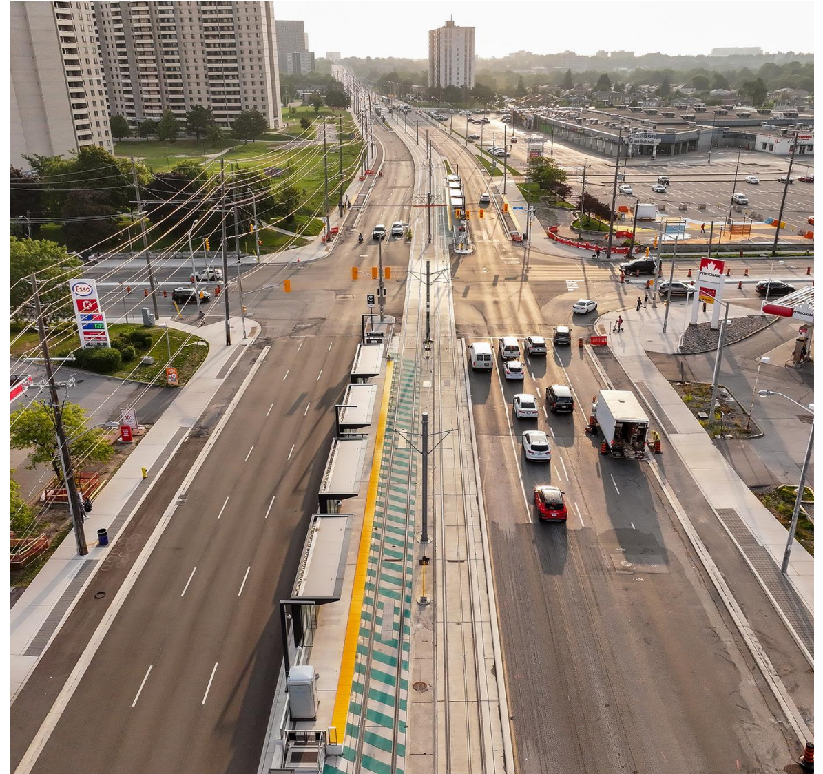
Photo: Finch West Avenue and Jane St. east aerial view 2024.08.24
