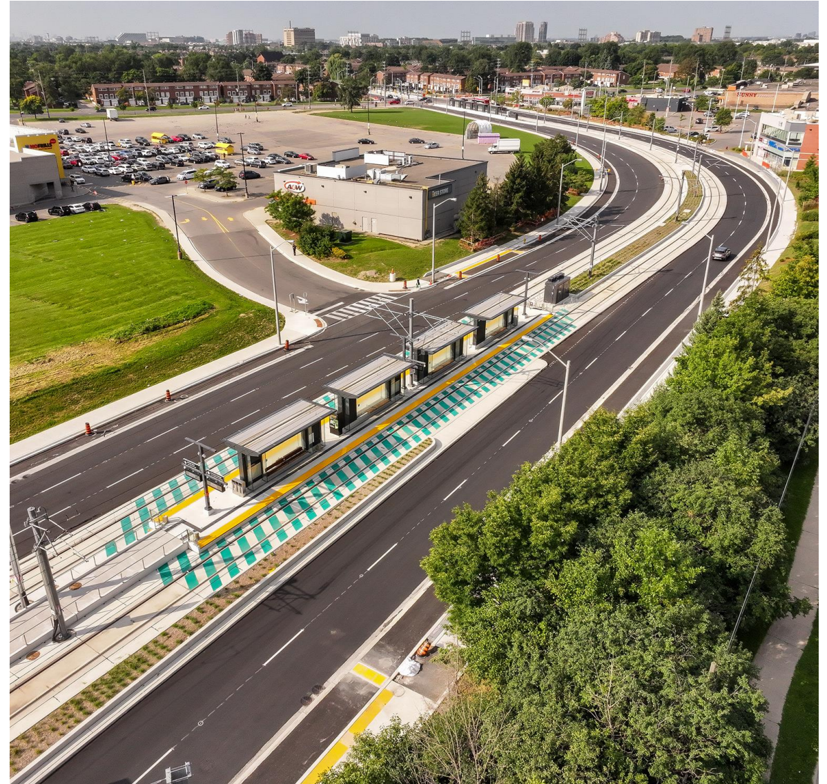
Photo: Finch Avenue West at Stevenson Stop, aerial view southwest. 2024.08.24
