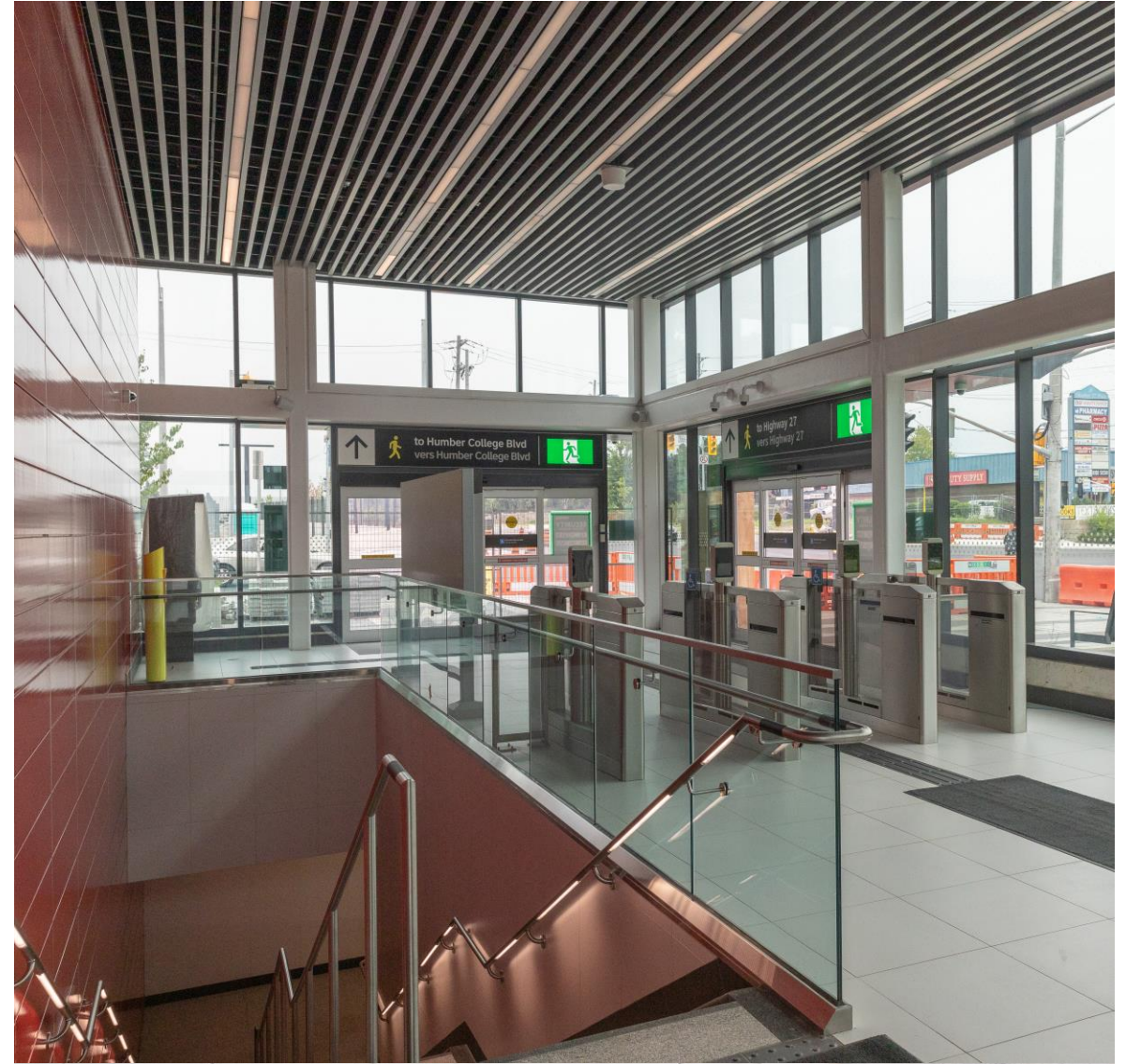
Photo: Humber College station exterior south building. 2024.06.31
