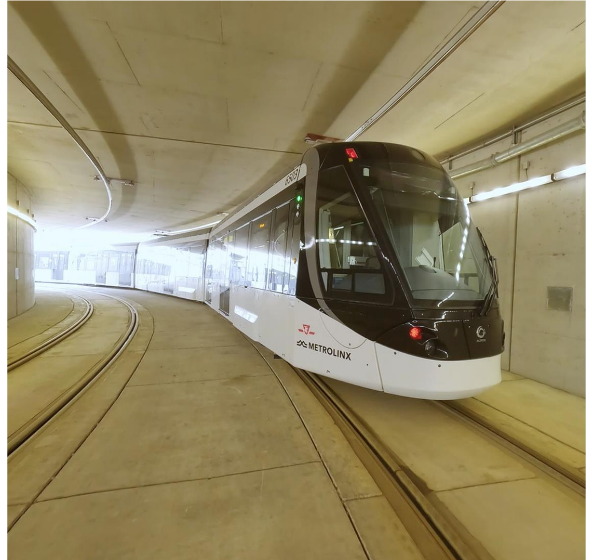
Photo: A Light Rail Vehicle travels through the Humber College portal. 2024.03.08
