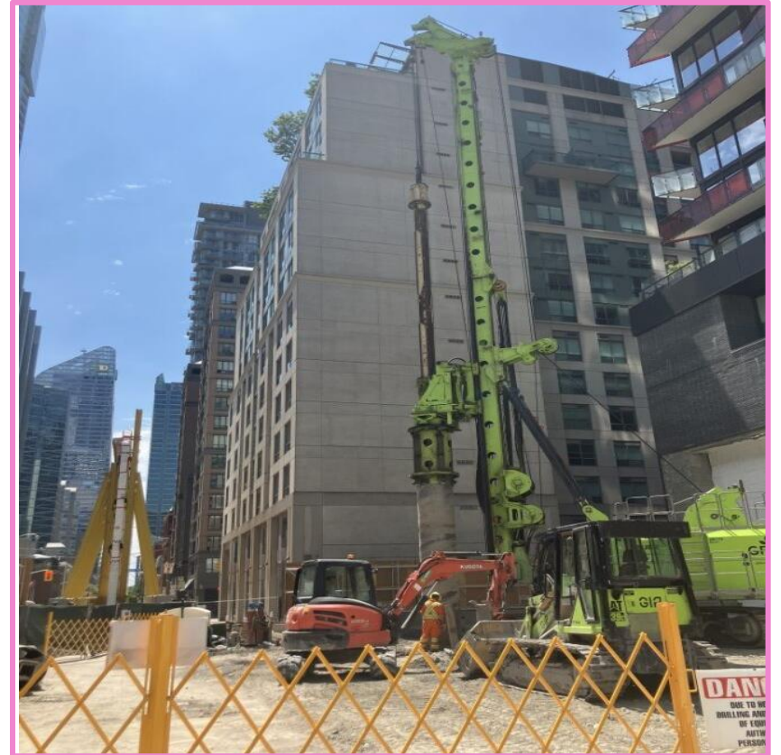
Piling machine at the South site
