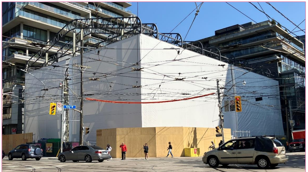
King-Bathurst north site acoustic shelter, where excavation work will occur.
