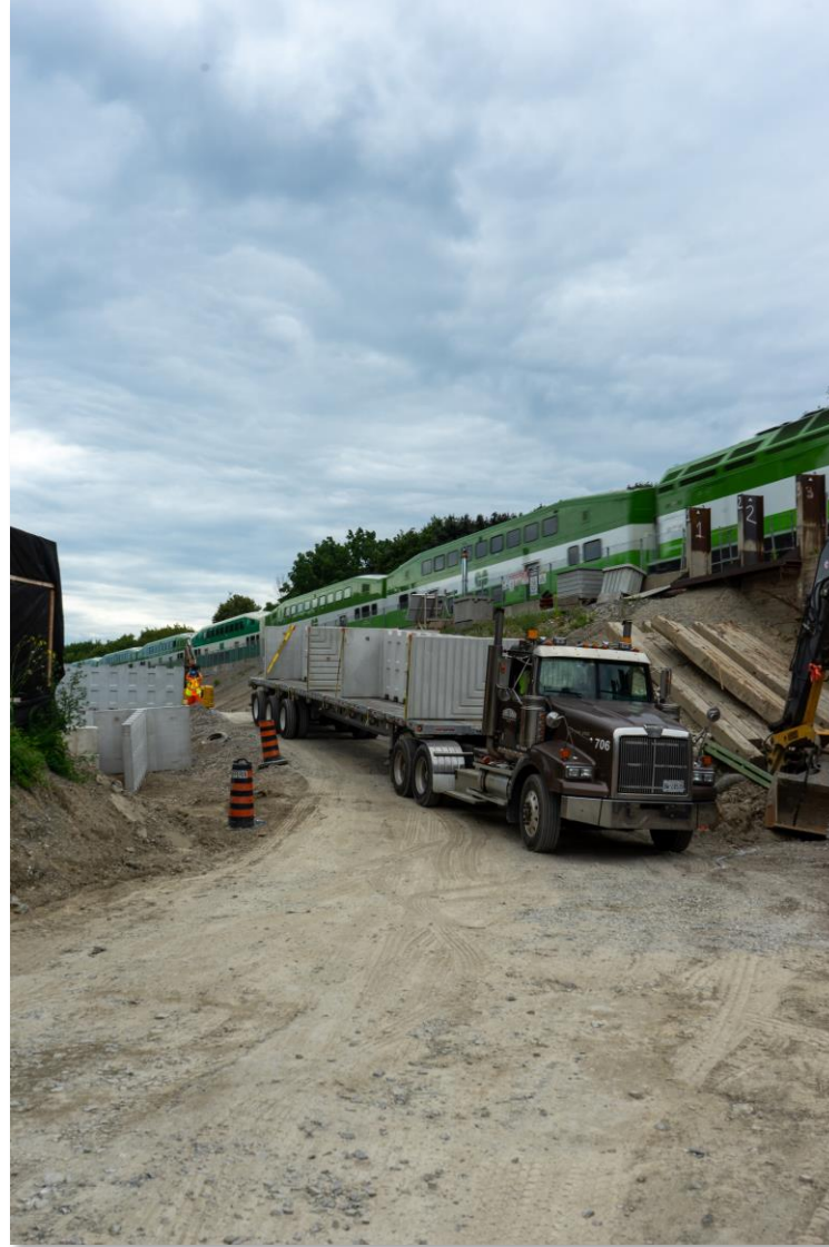
Delivery of t-blocks at Dundas St. E.
