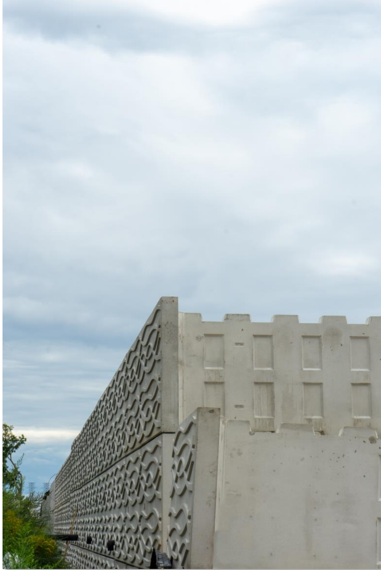
Emerging design on installed t-block south of Queen St. E.
