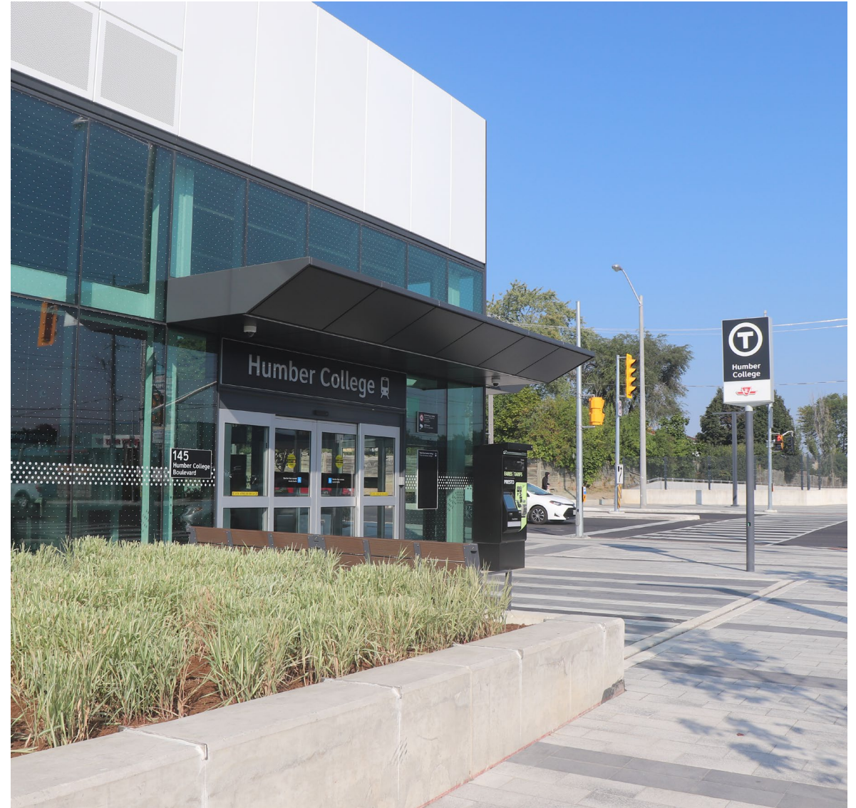
Photo: Humber College station exterior south building. 2024.09.20
