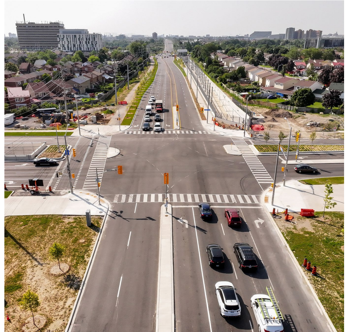
Photo: Highway 27 and Finch Avenue West, aerial view south. 2024.08.24
