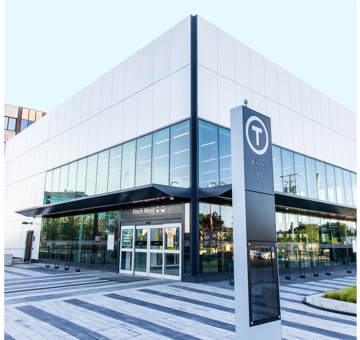
Photo: Finch West LRT station pedestrian concourse. 2024.08.24
