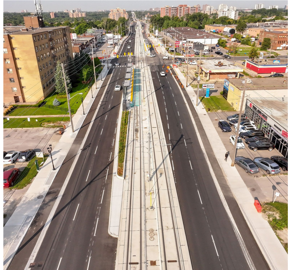
Photo: Finch Avenue West and Milvan Drive, aerial view west. 2024.08.24
