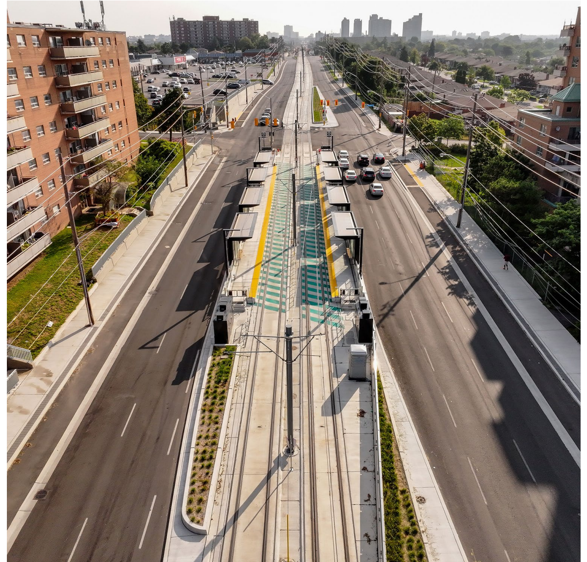
Photo: Finch Avenue West and Pearldale Avenue, aerial view west. 2024.08.24
