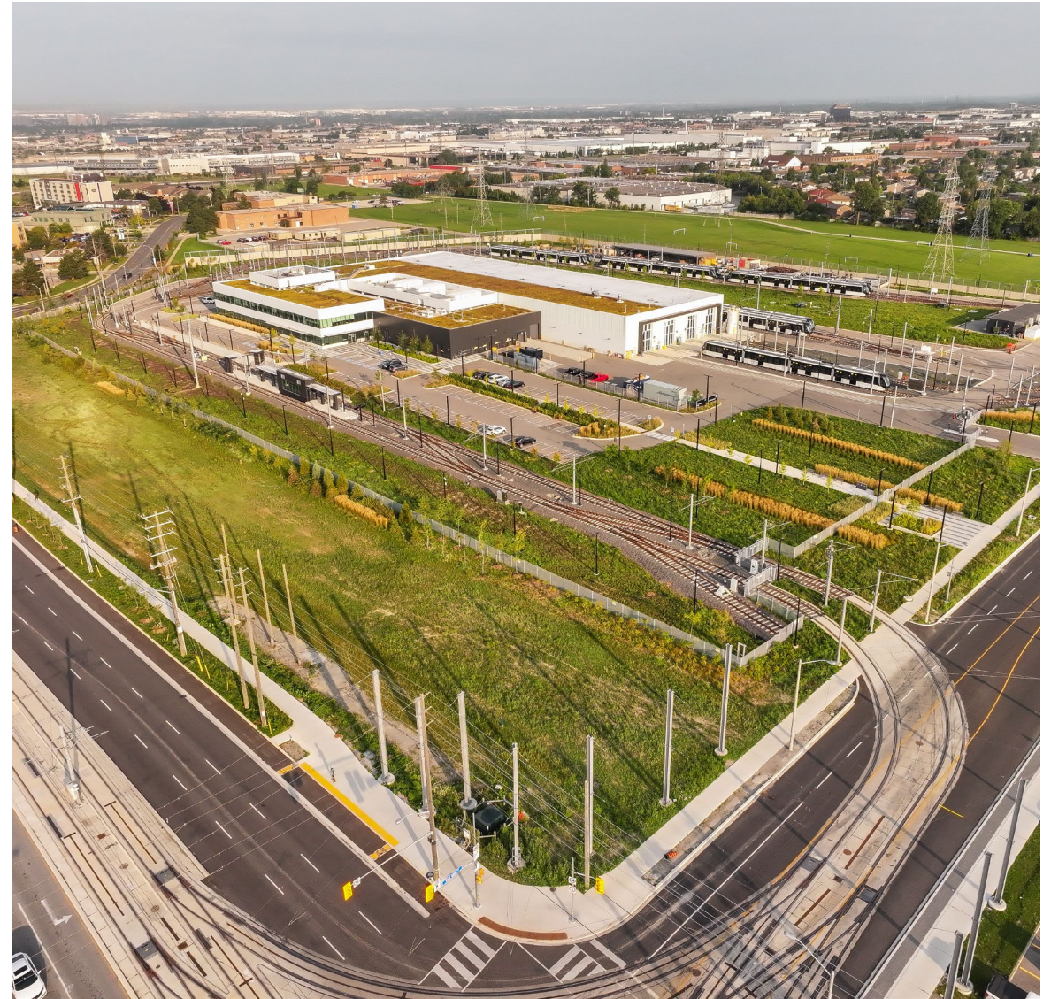
Photo: Maintenance and Storage Facility, northwest aerial view. 2024.08.24
