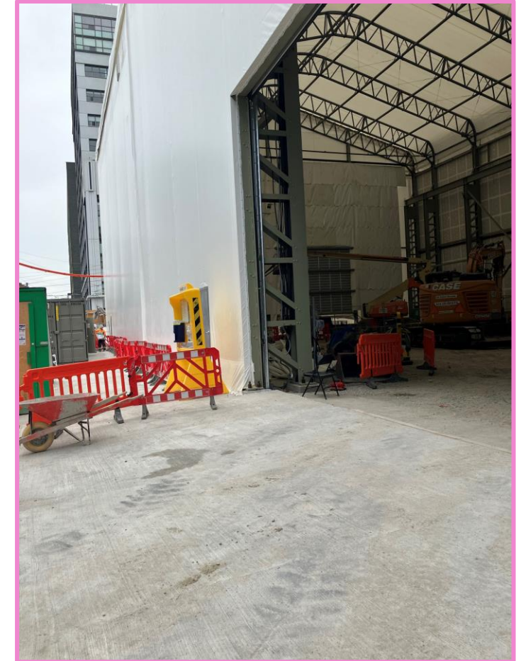
Paved worksite to reduce dust.
