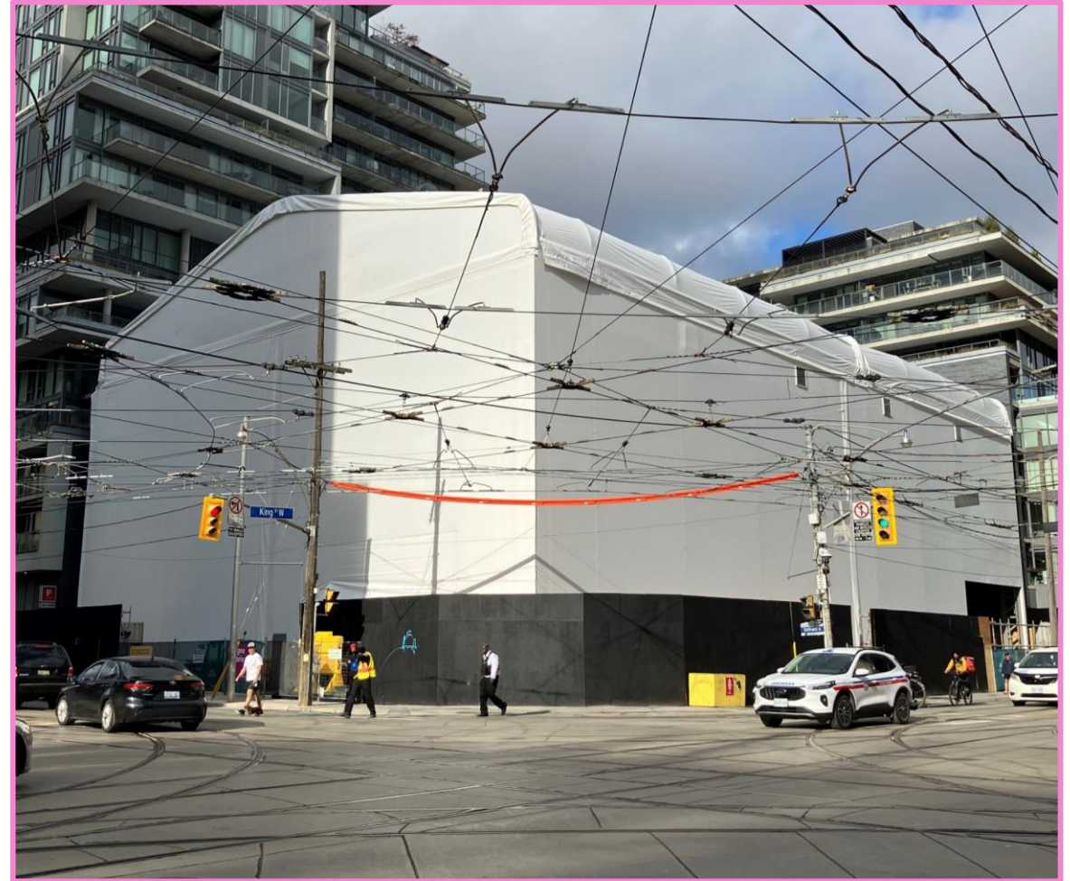
Current installation works of the acoustic shelter exterior canvas.
