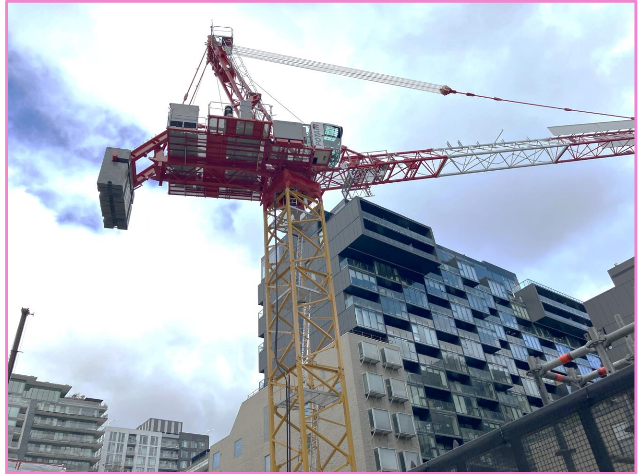
Tower crane installed at King-Bathurst (south).
