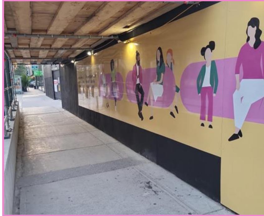
Protective hoarding surrounding the south site.
