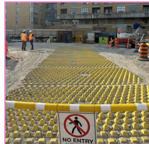
Example of mud mat installed
