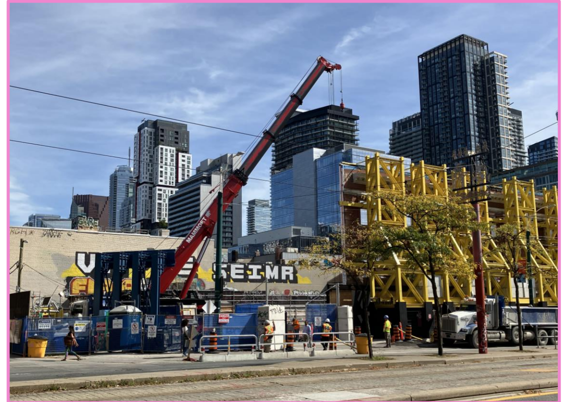
Crane installation at Queen-Spadina North site
