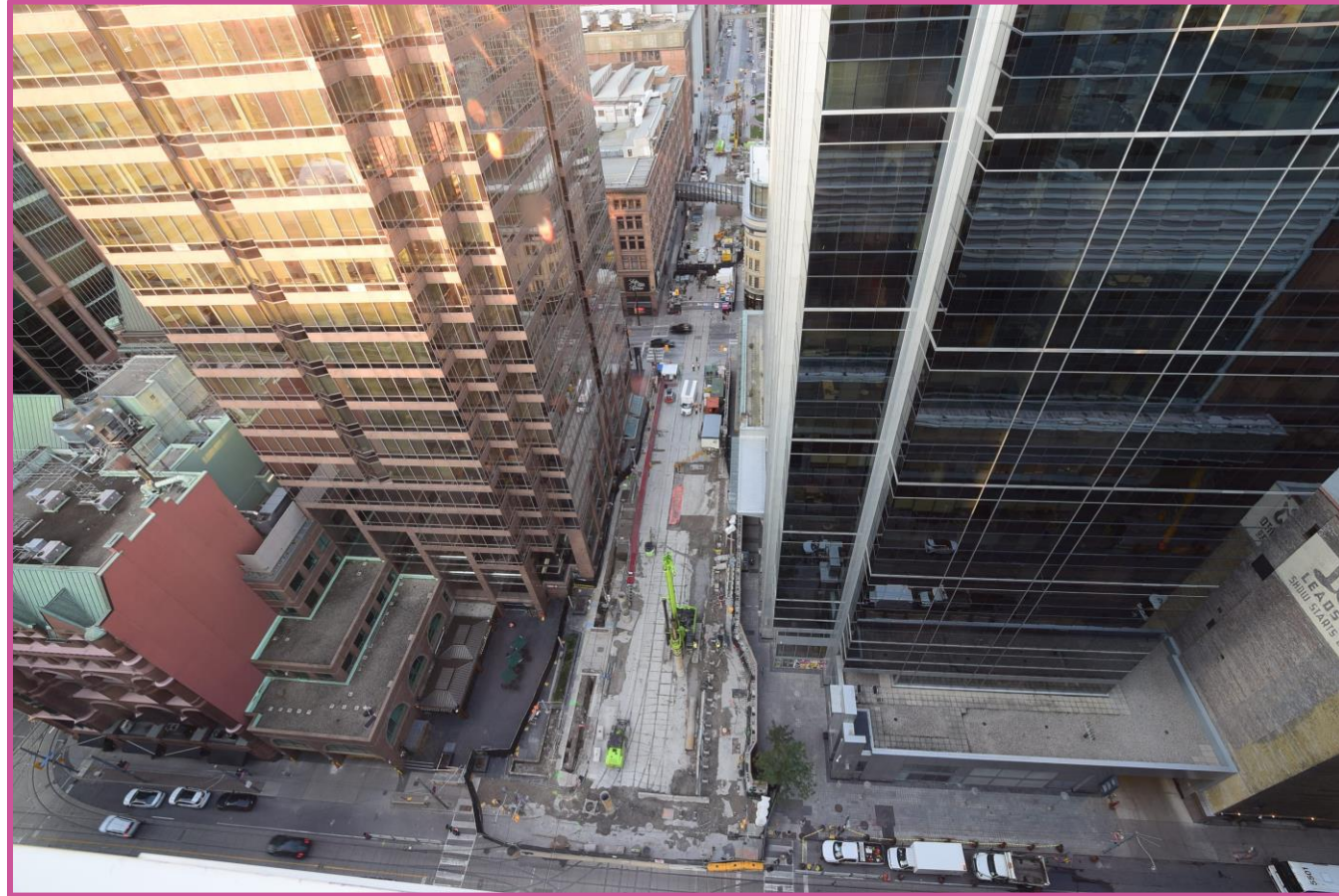
Work progress at the West site - October 2024
