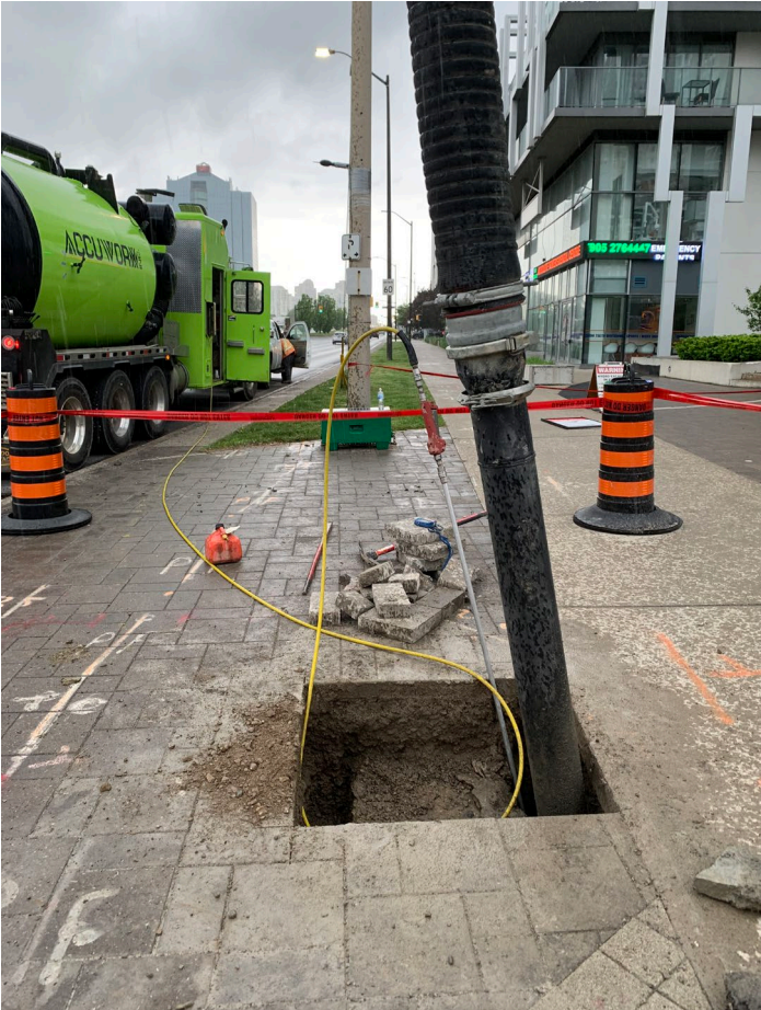
Subsurface Utility Engineering (SUE)
