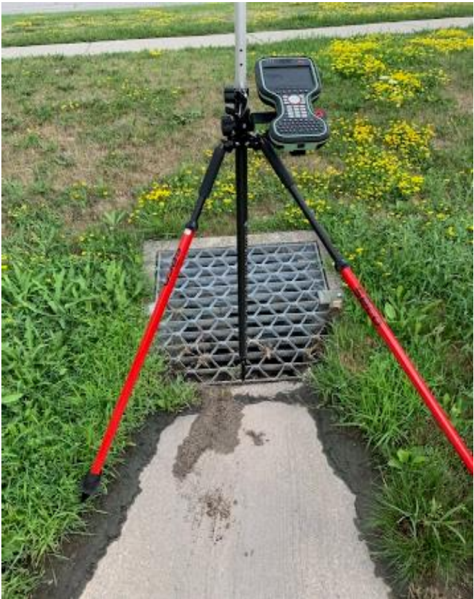
Subsurface Utility Engineering (SUE)
