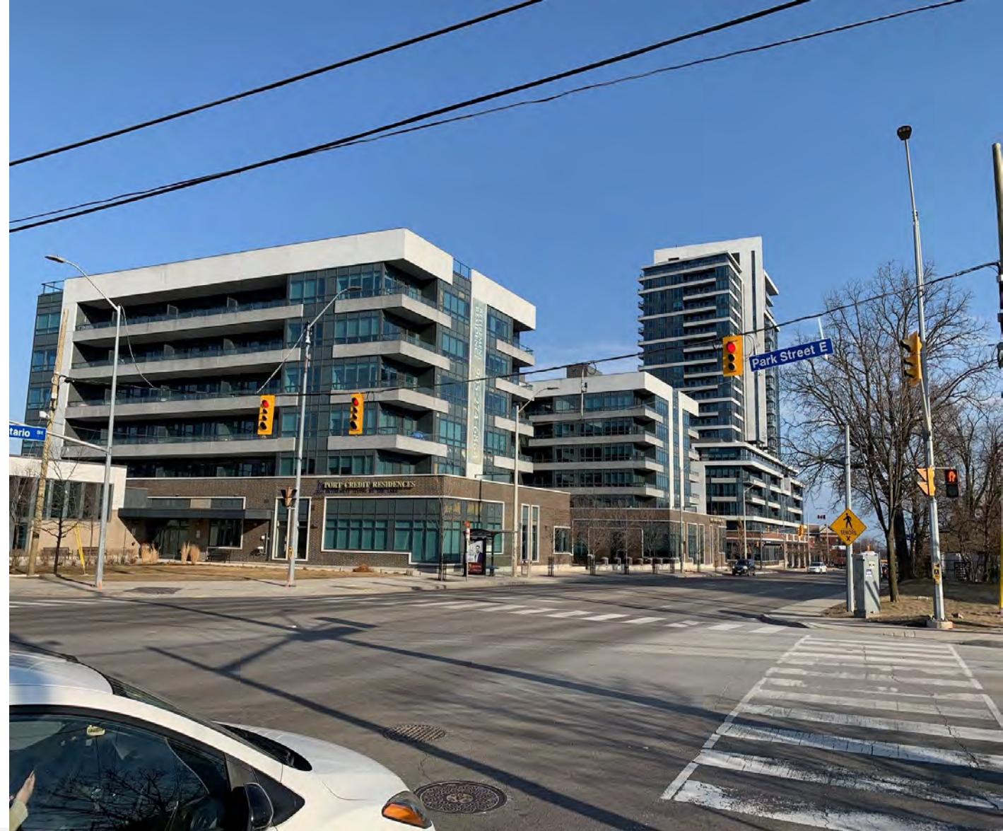
Temporary Traffic Signals
