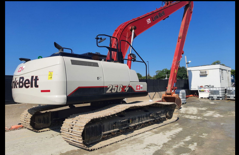
Sanitary infrastructure relocations-Mississauga North
