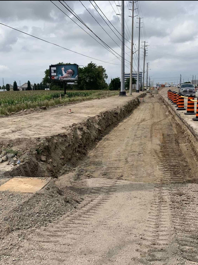
Road widening-Mississauga North
