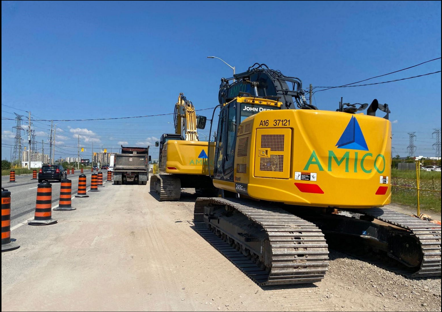
Stormwater infrastructure relocations-Mississauga North
