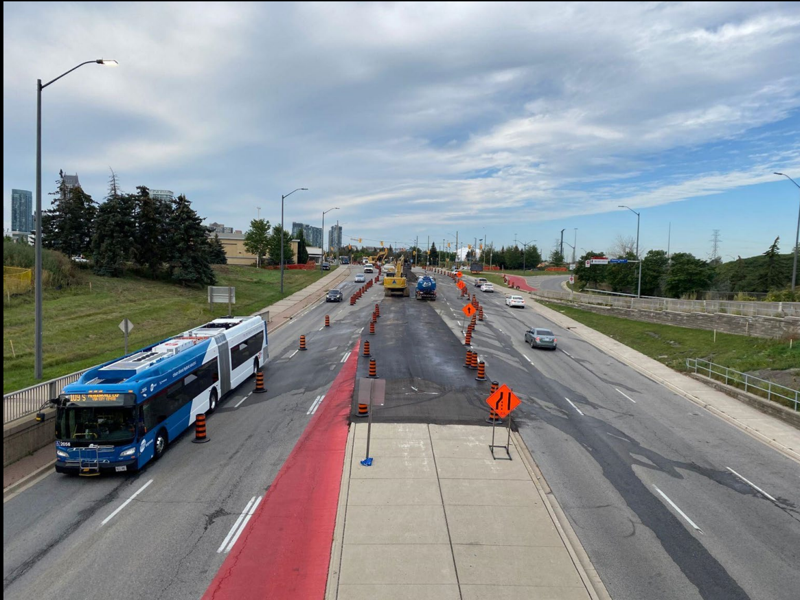
Utility relocations begin on Rathburn Road-Mississauga Centre
