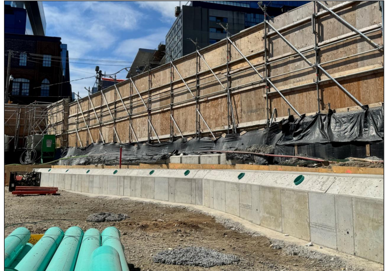
Capping beam ready for tie-back supports near King St E
