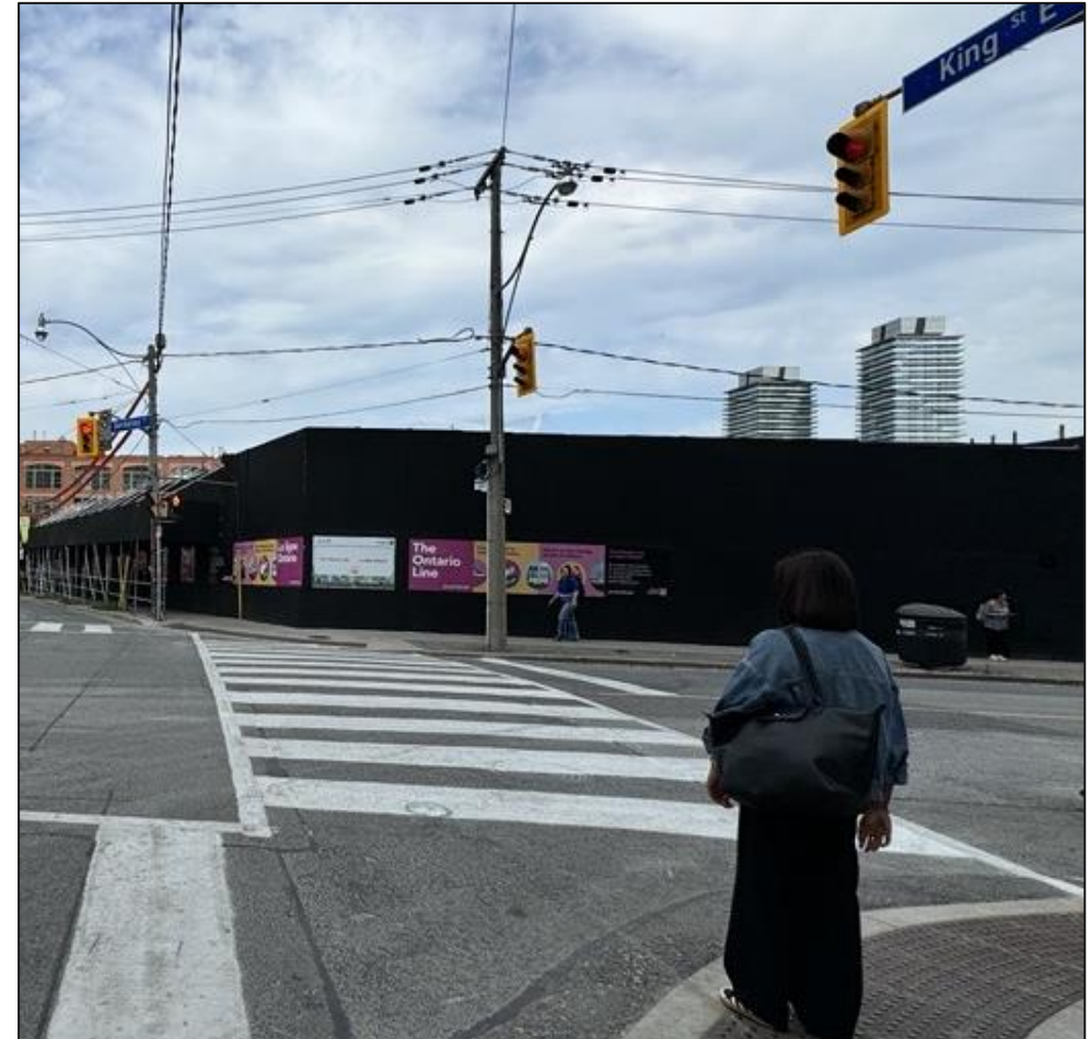
5 metre noise wall at King St E and Berkeley St
