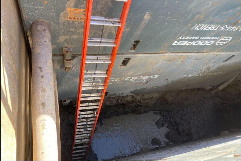
Sanitary infrastructure relocations in Mississauga Centre
