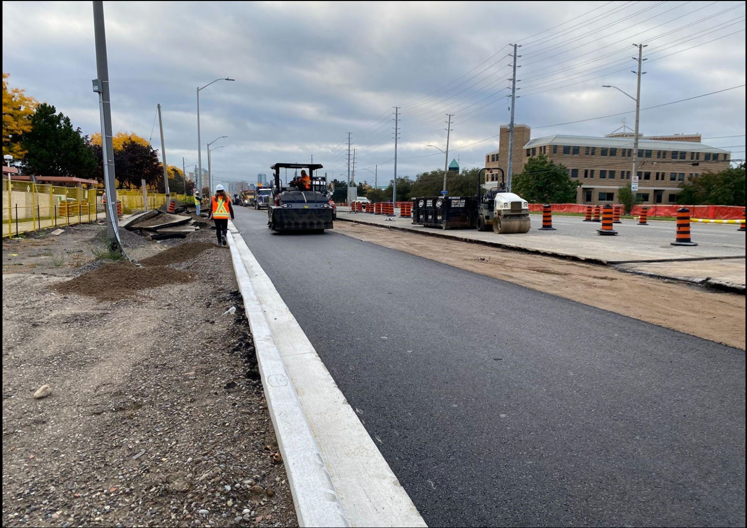
Road Widening in Mississauga North
