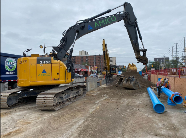
Watermain Installation in Cooksville
