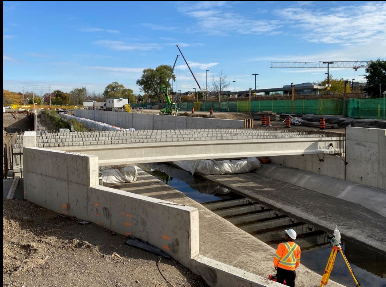
Floodwall and Pedestrian Bridge Construction at Mary Fix Creek
