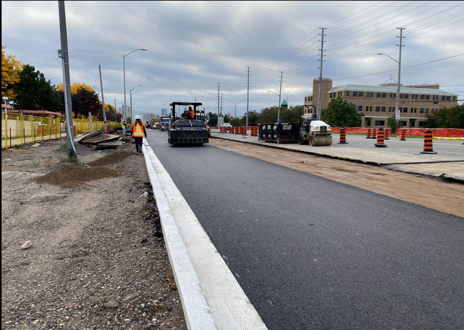
Road Widening in Mississauga North
