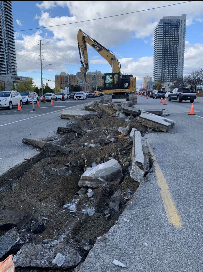
Remaining Median Removals in Mississauga North
