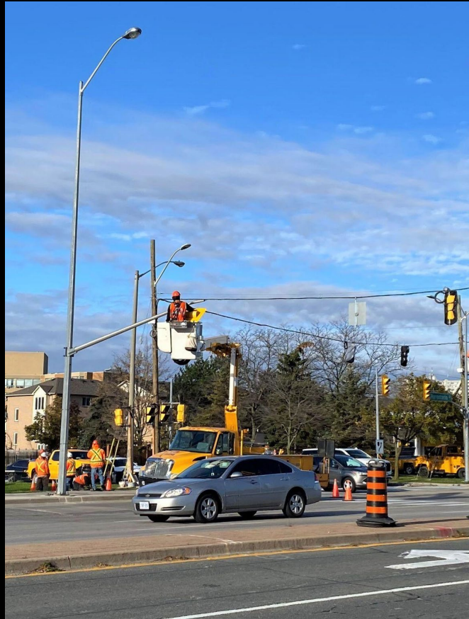
Temporary Traffic Signal Installations in Brampton South
