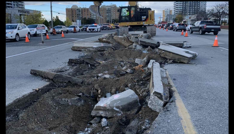
Removal of Remaining Medians in Mississauga North
