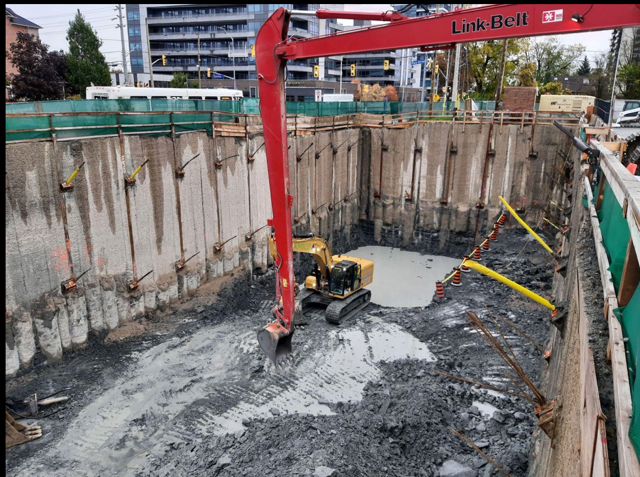
Construction of the LSW Push Box and Excavation to Service Level at Port Credit GO LRT Station
