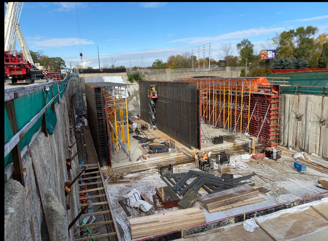
Construction of the LSW Push Box and Excavation to Service Level at Port Credit GO LRT Station
