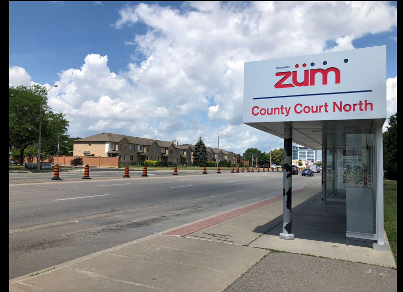
Staging for Median Removals in Brampton South
