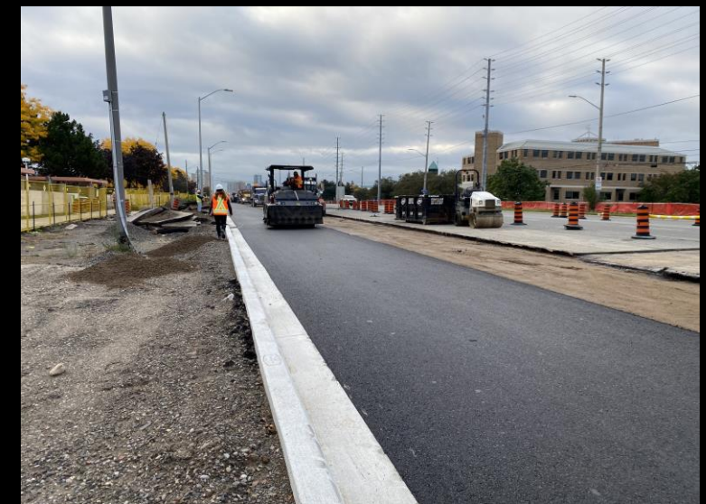
Road Widening –Mississauga North
