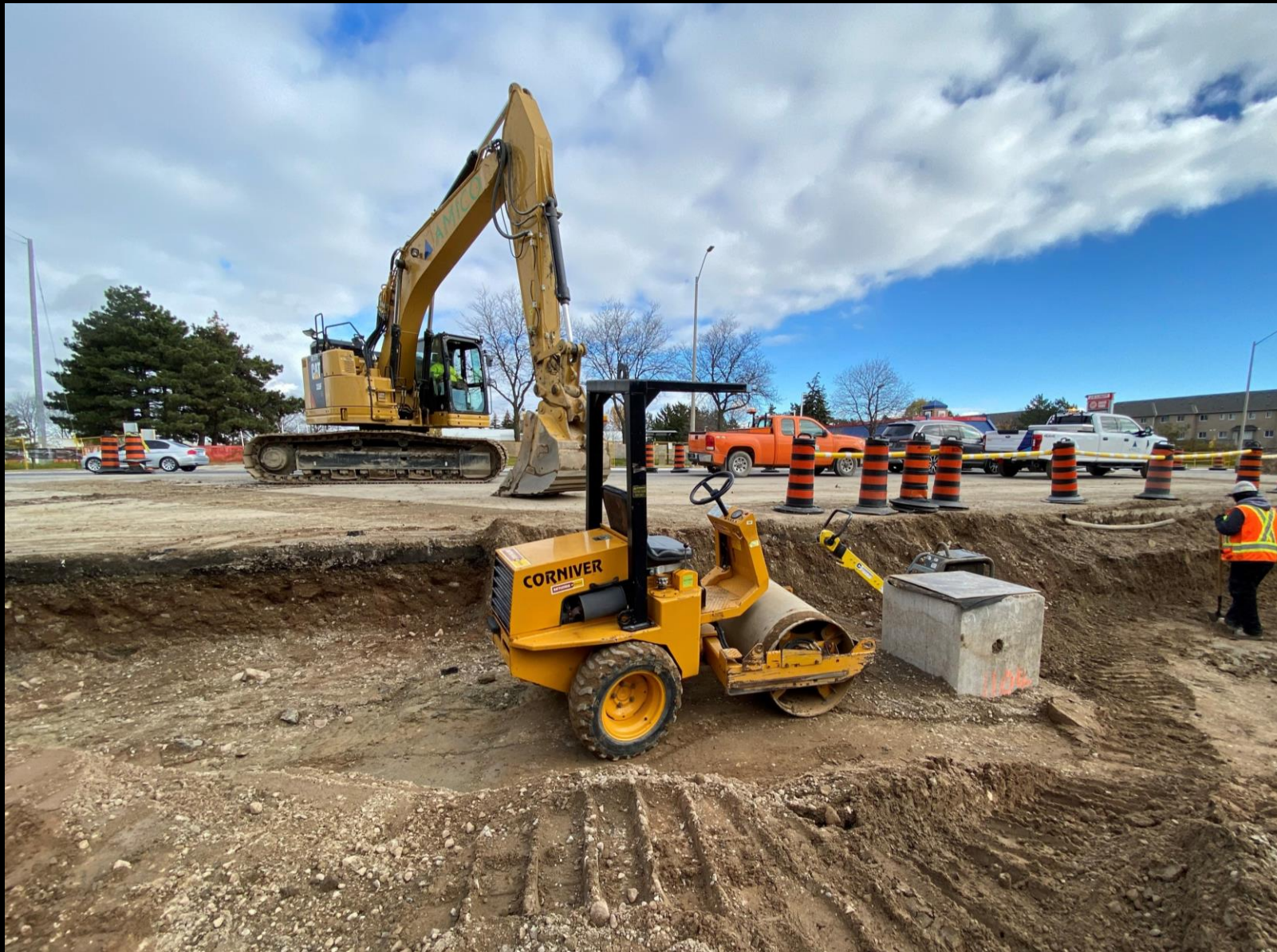
Road Widening – Mississauga North
