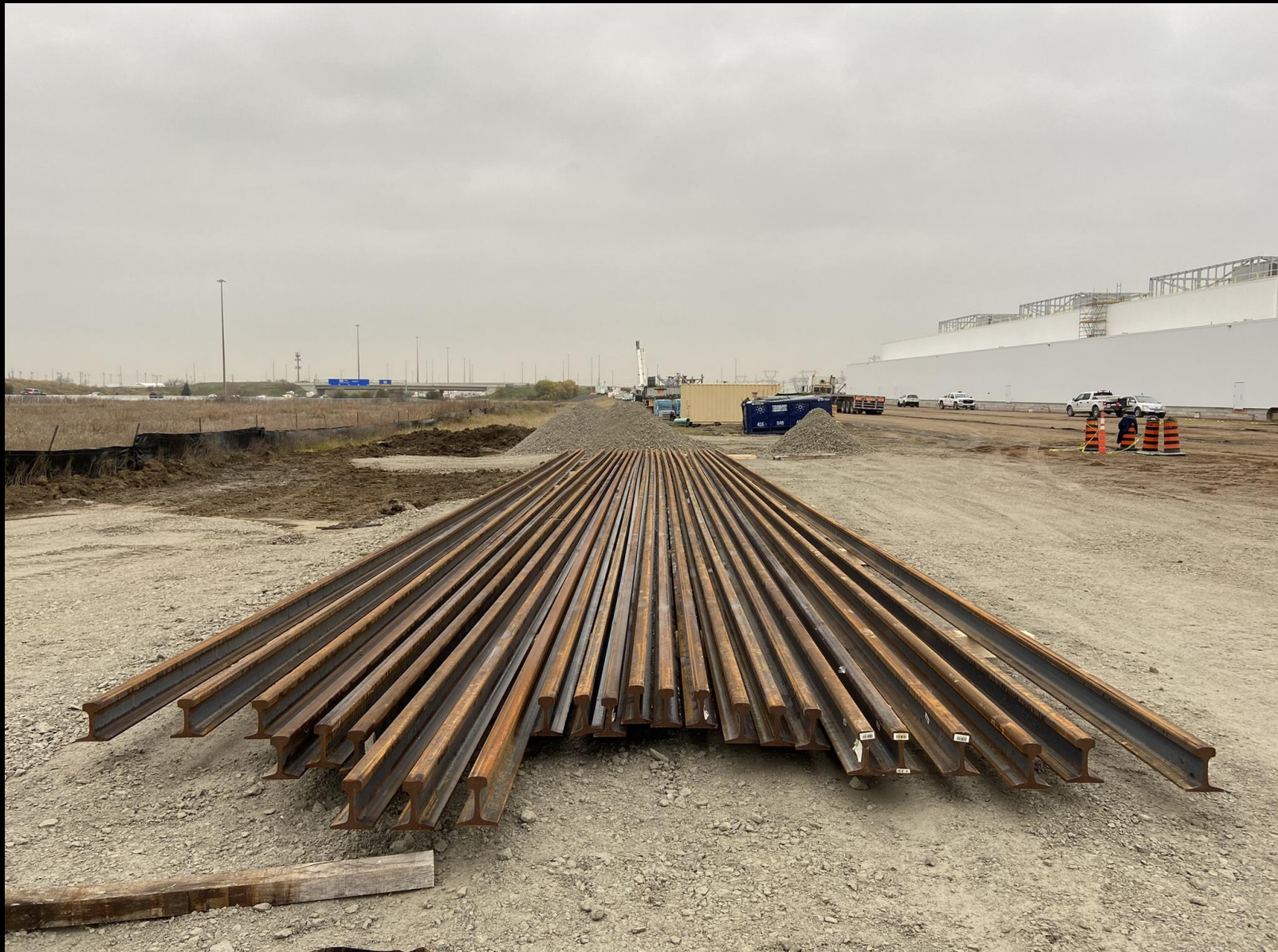
3000 m of Rail Delivered to the OMSF
