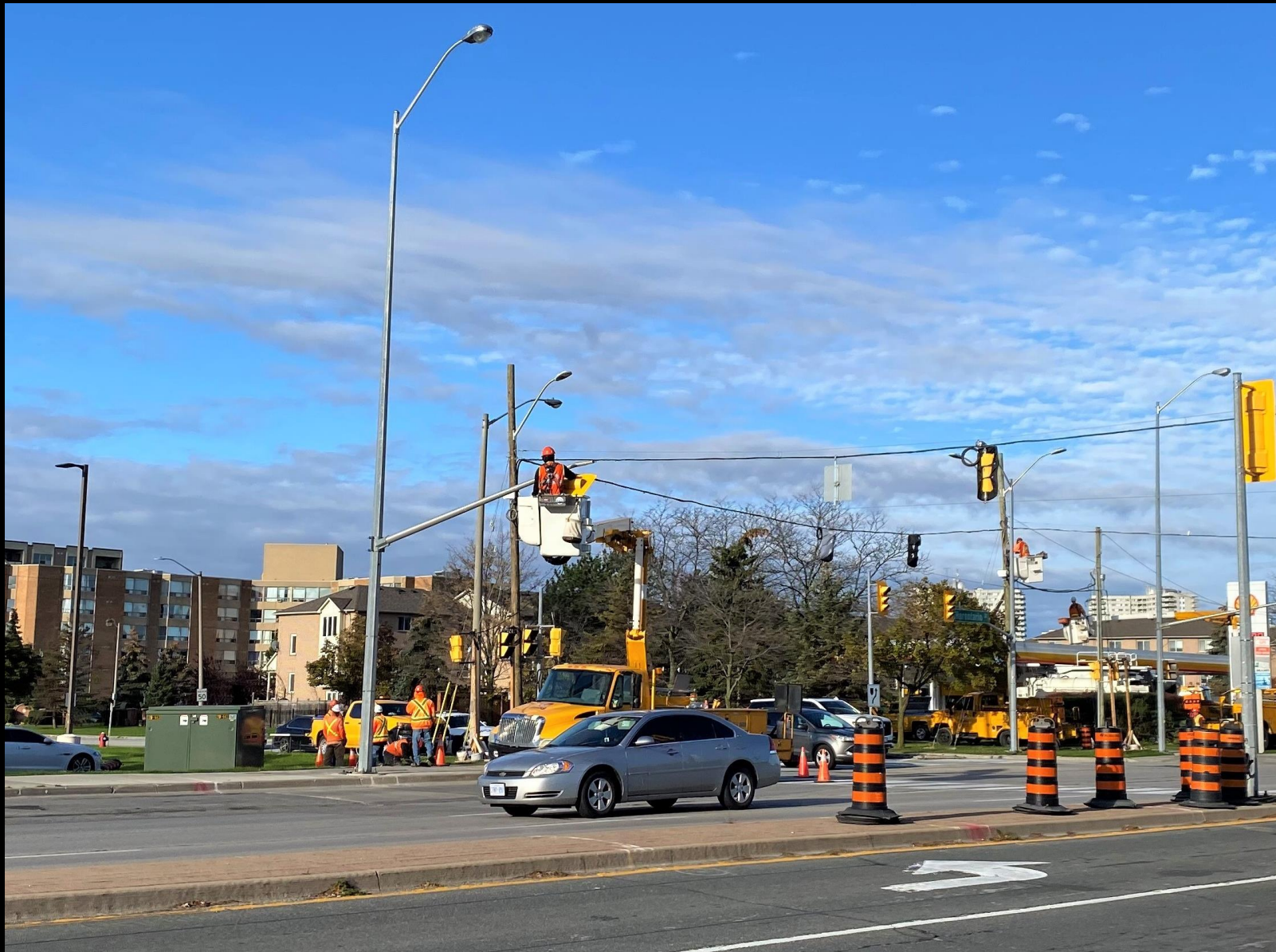
Temporary Traffic Signal Installation – Brampton South
