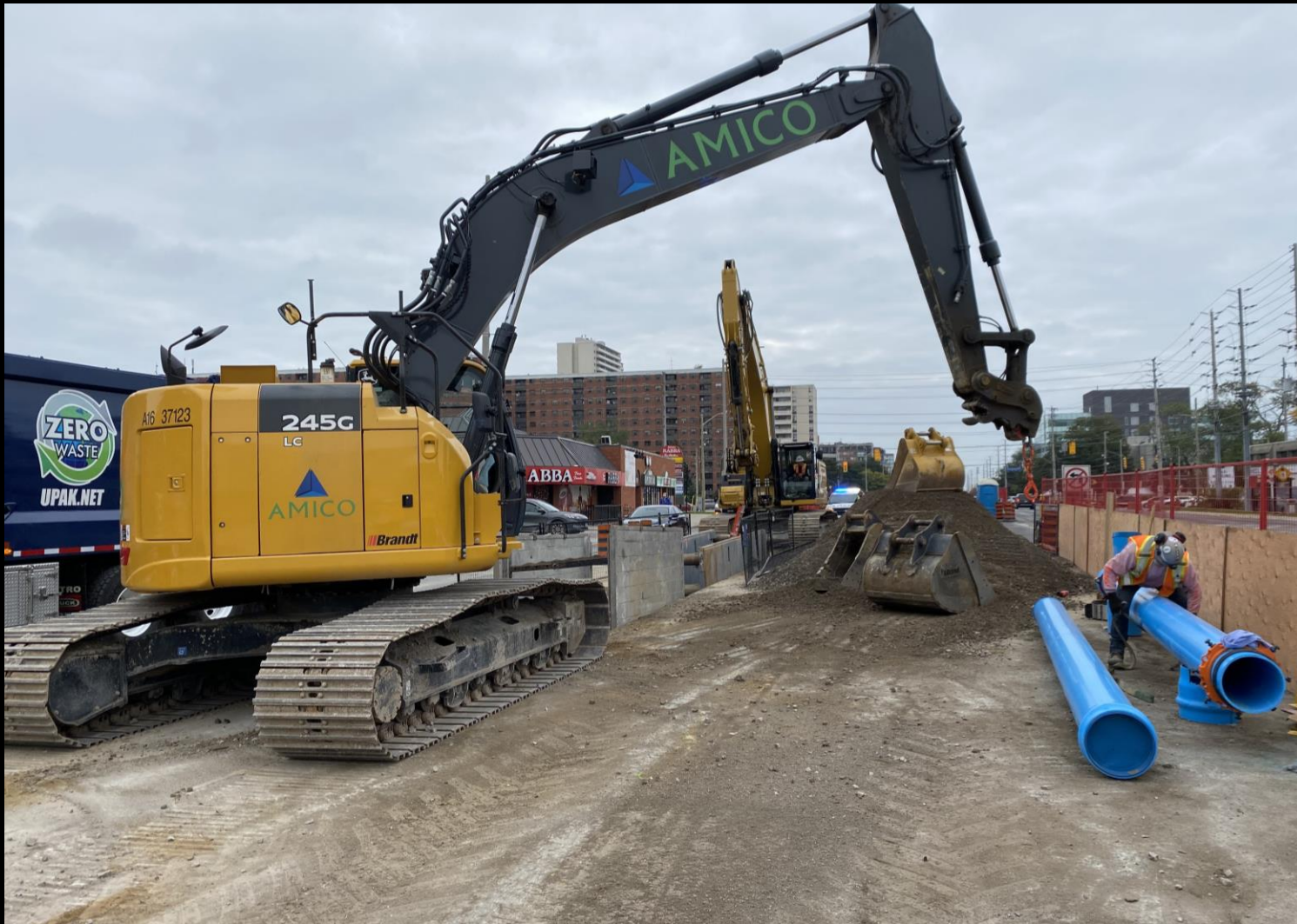
Watermain Installations - Cooksville
