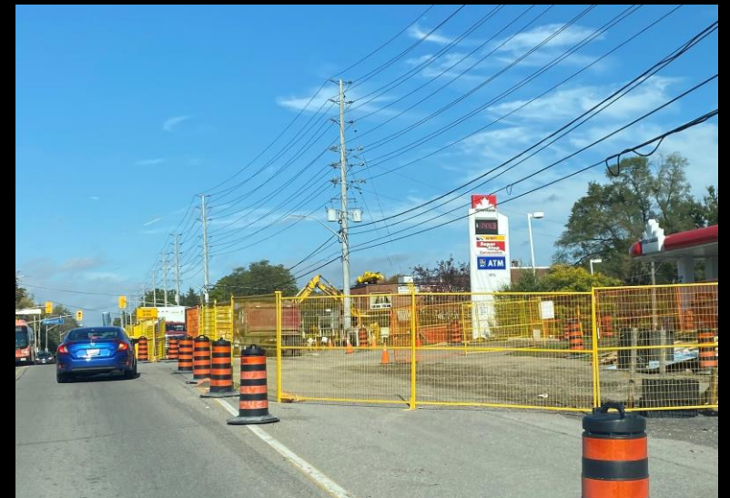
Dry Utility Alectra Works –Mississauga South
