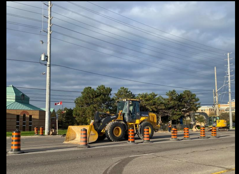
Road Widening – Mississauga North
