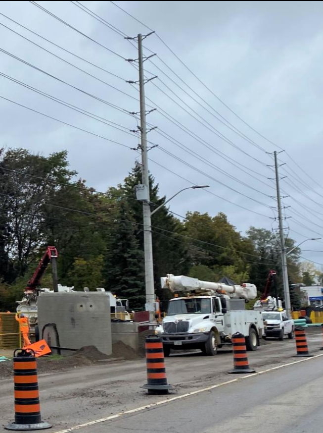
Dry Utility Alectra Works -Mississauga South
