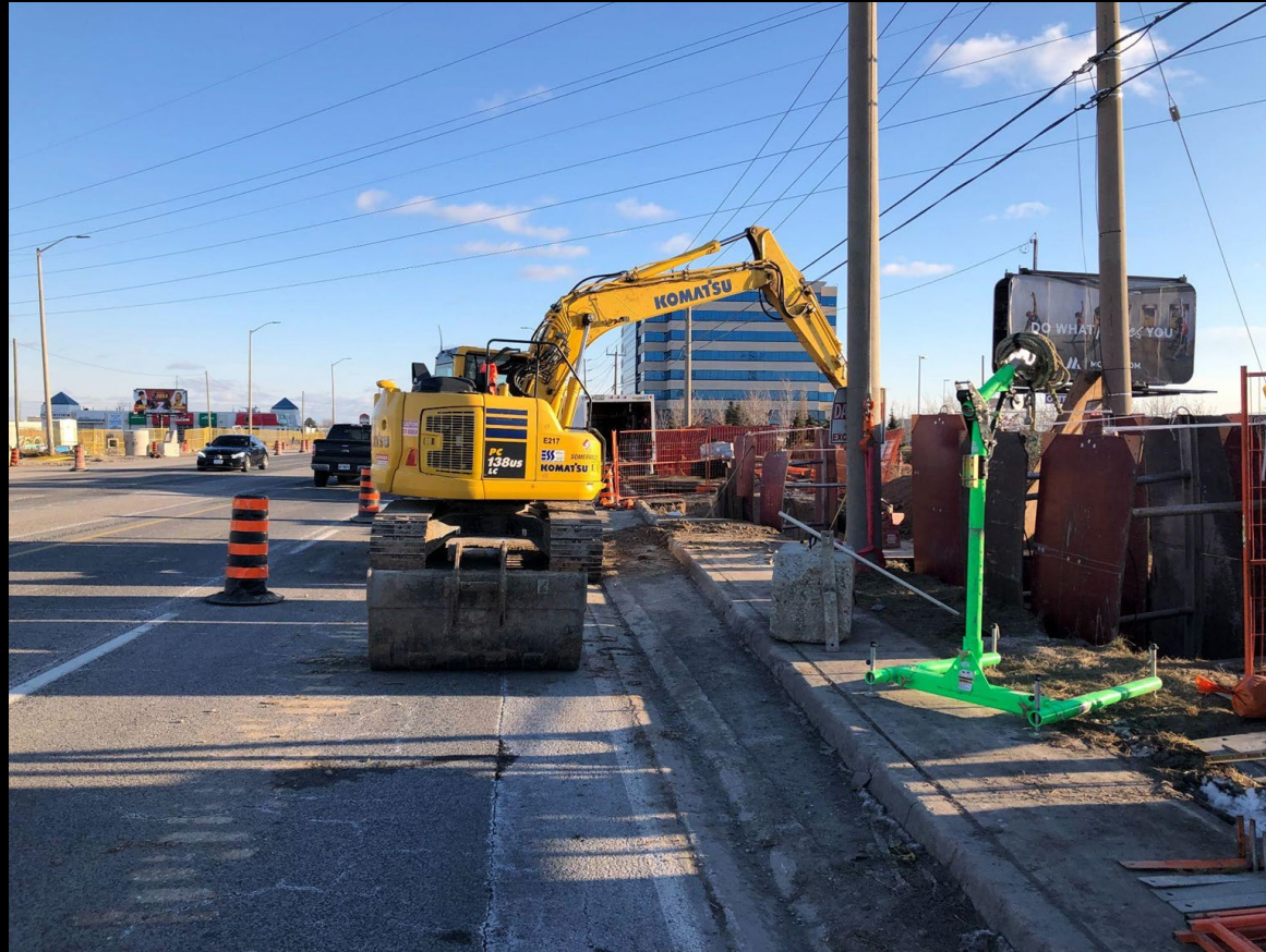
Utility Relocations in Mississauga North
