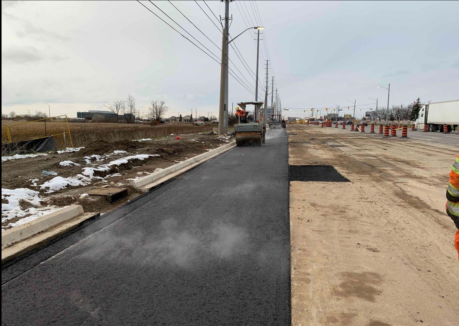
Road Widening in Mississauga North
