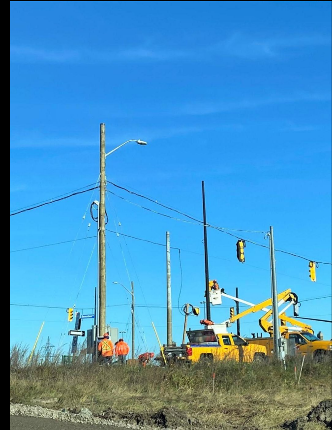
Temporary Traffic Signal Installations in Mississauga Centre
