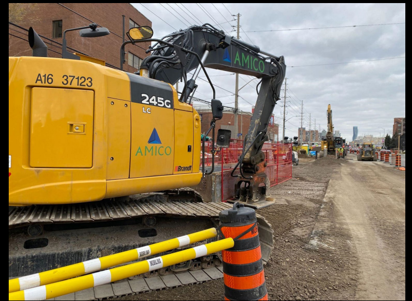
Water Main Installation in Cooksville
