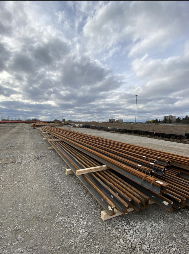
Delivery of Rails to OMSF in Brampton South
