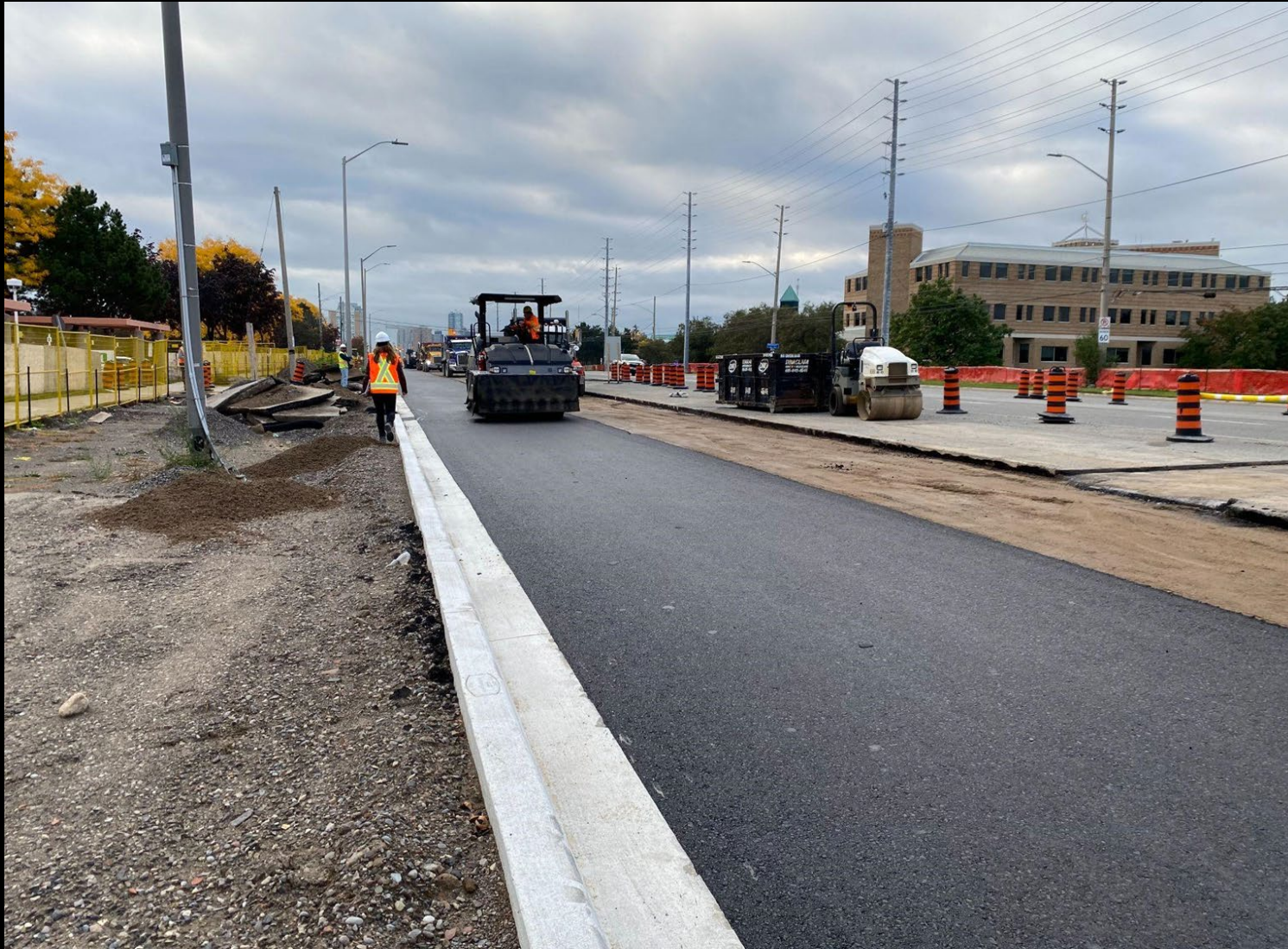
Road widening in Mississauga North
