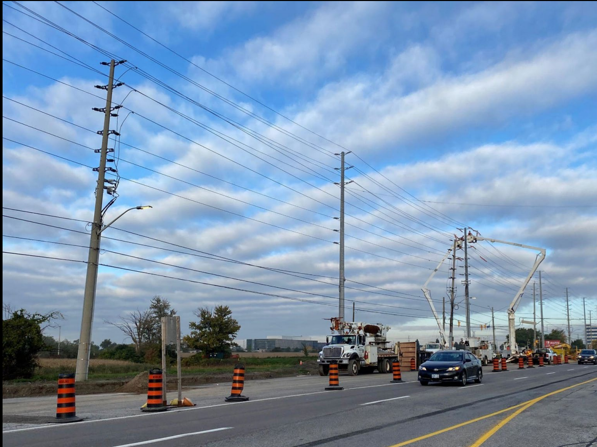
Dry utility relocations in Mississauga North
