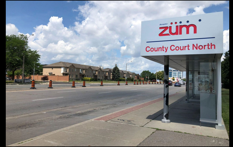
Staging for median removals in Brampton South
