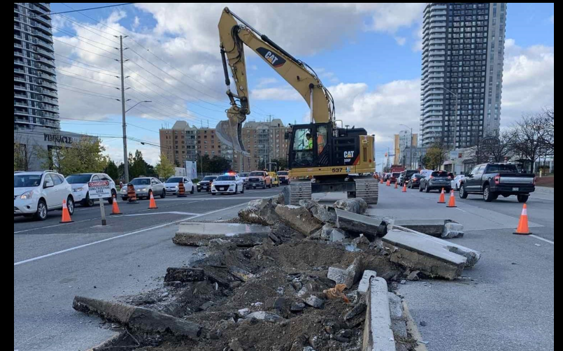
Removal of remaining medians in Mississauga North
