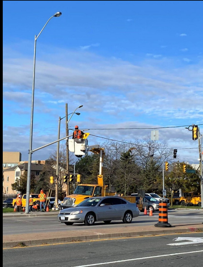
Temporary traffic signal installations in Brampton South
