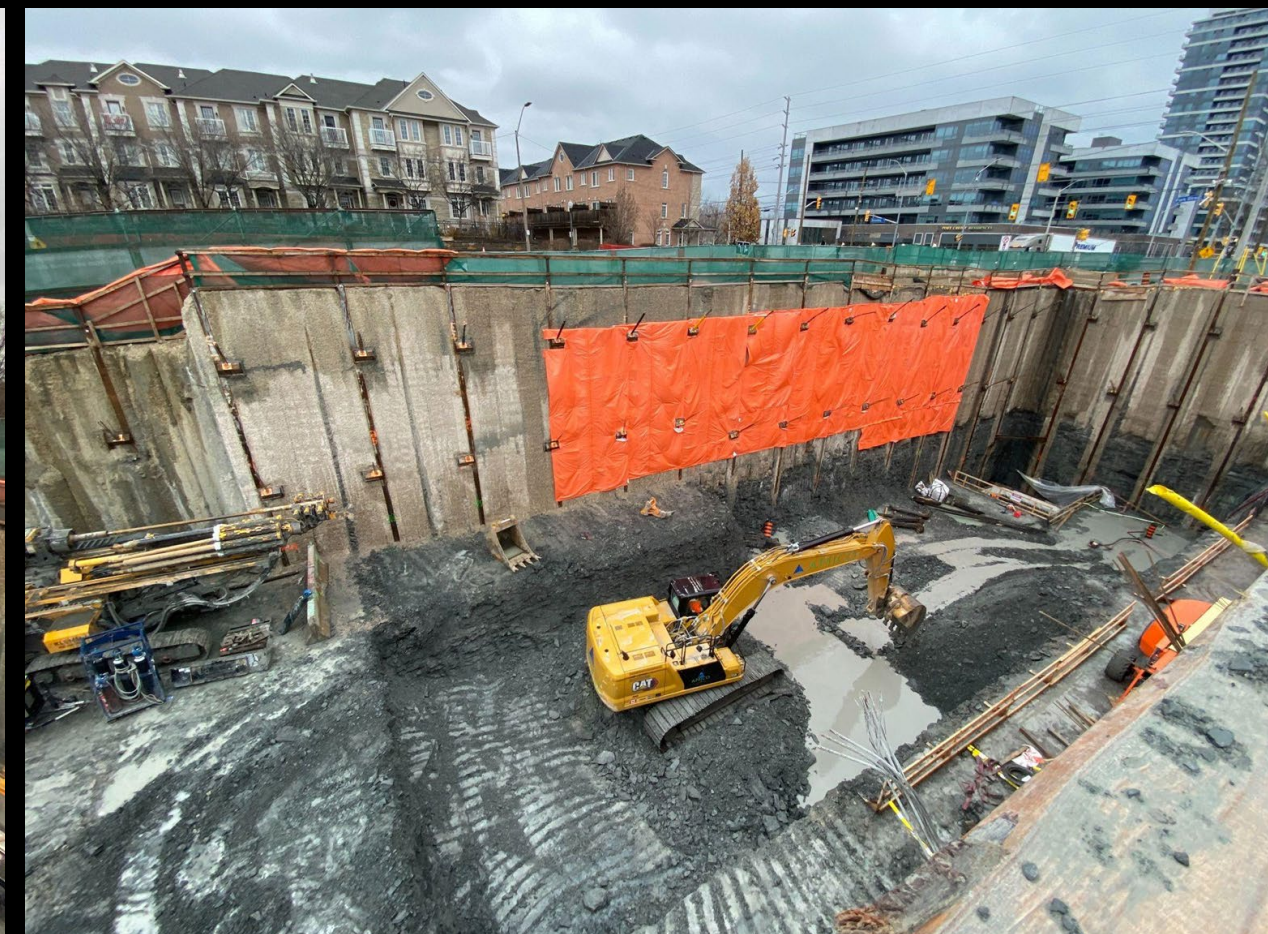
Port Credit Station - Excavation
