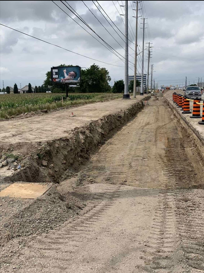
Road widening-Mississauga North
