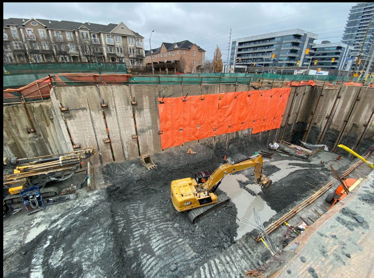
Port Credit Station - Excavation
