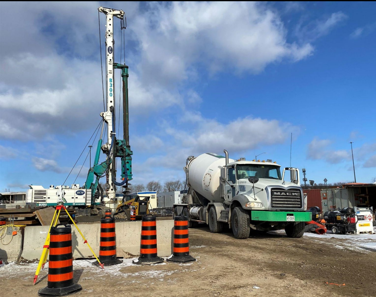
Caisson Drilling for OCS Poles at the OMSF Facility in Brampton
