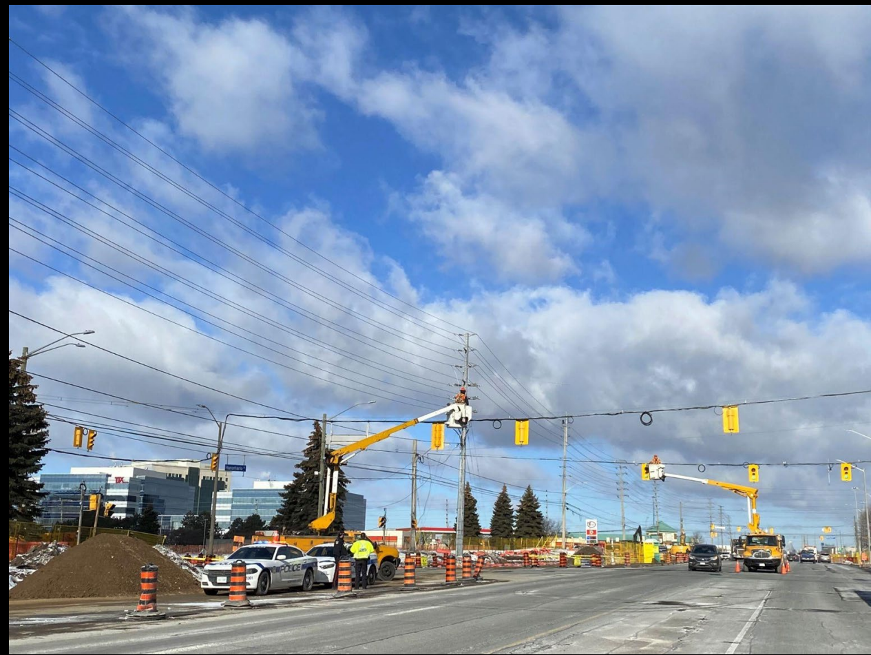
Temporary Traffic Signal Adjustments in Mississauga North
