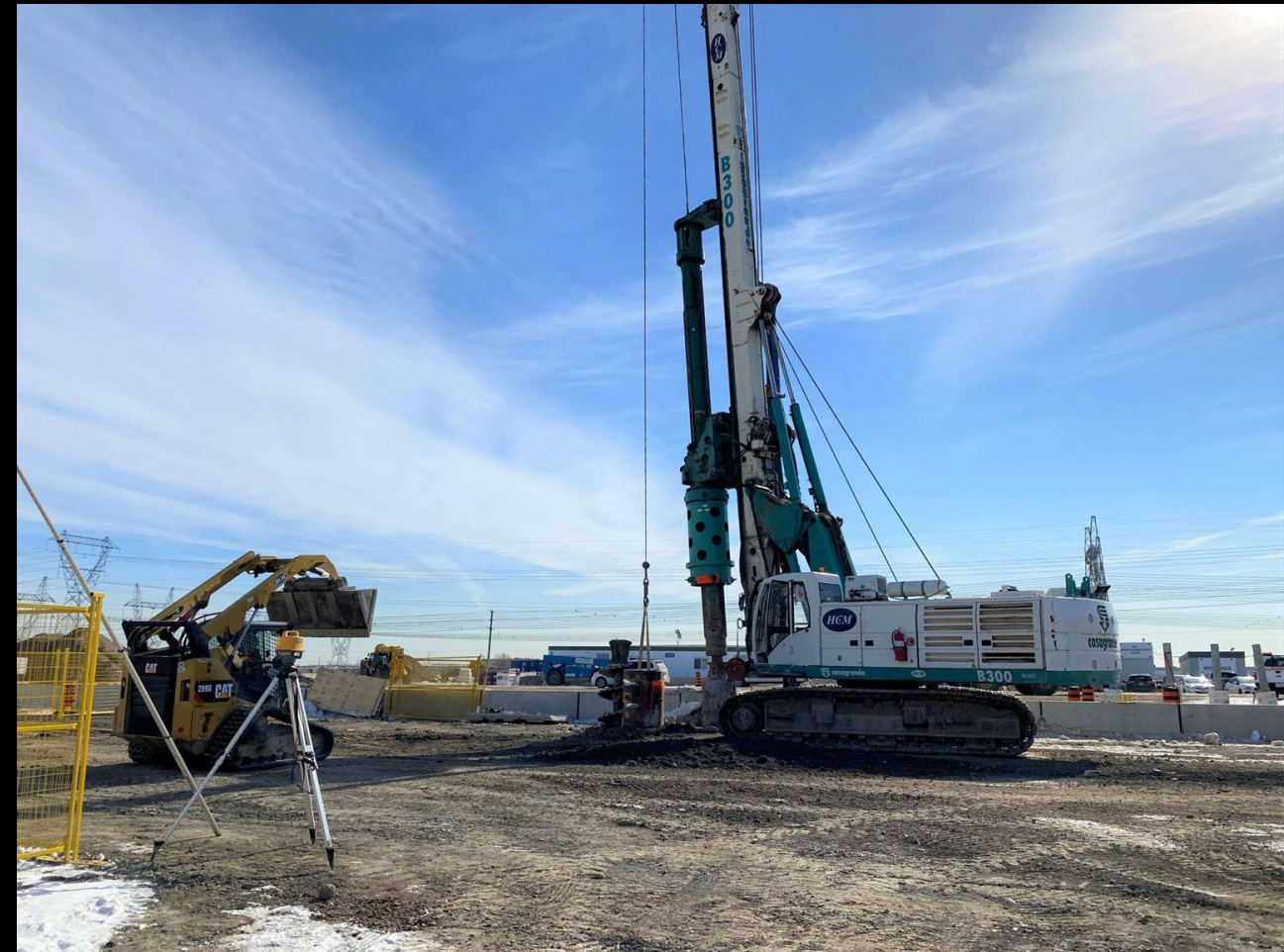
Caisson Drilling for OCS Poles at the OMSF Facility in Brampton
