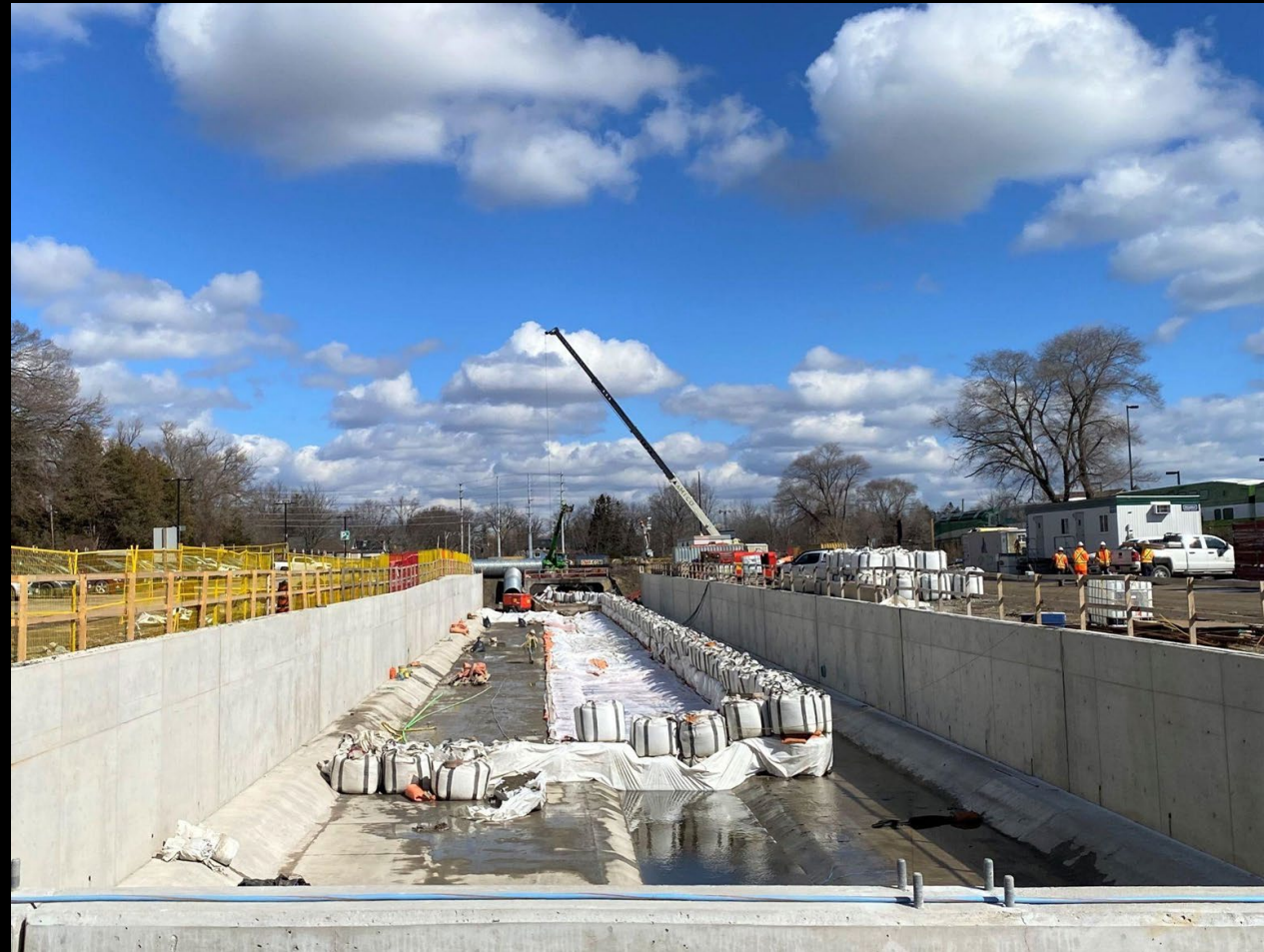
Mary Fix Creek - Channel Excavation
