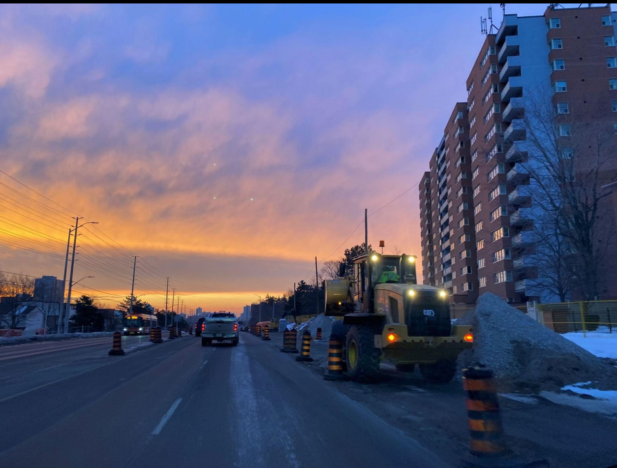
Utility Relocations in Cooksville
