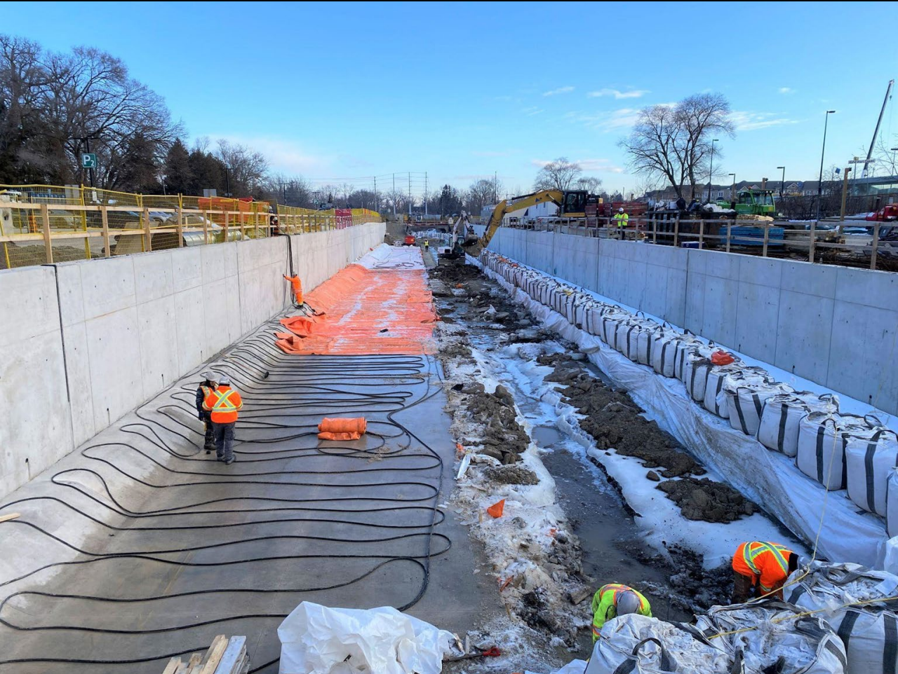
Mary Fix Creek - Channel Excavation
