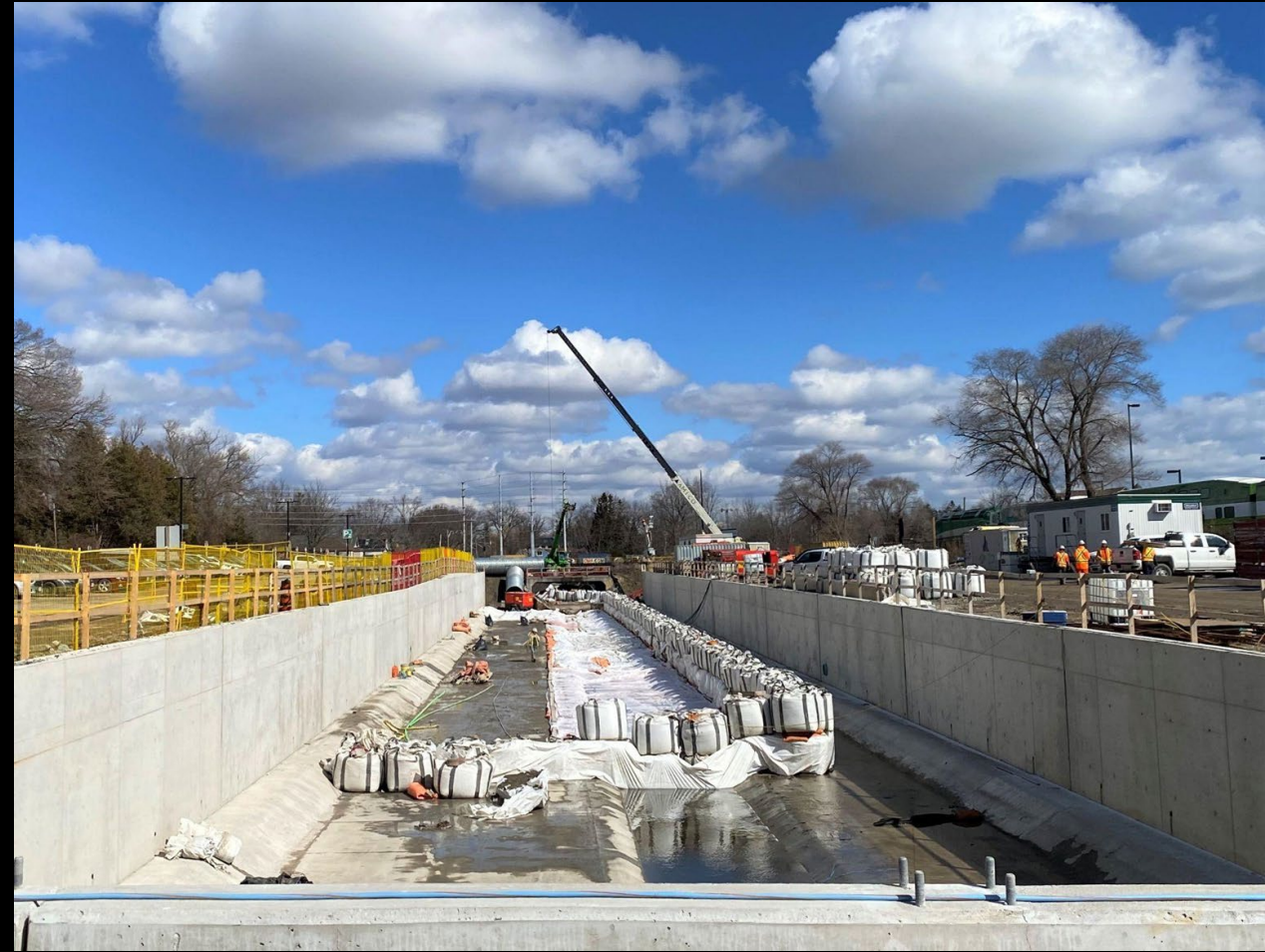
Mary Fix Creek - Channel Excavation
