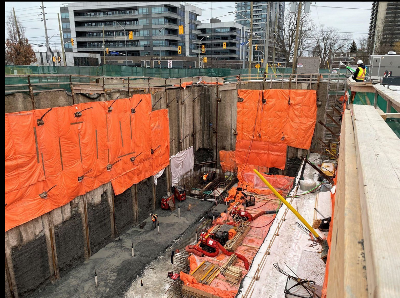
Port Credit Station - Excavation
