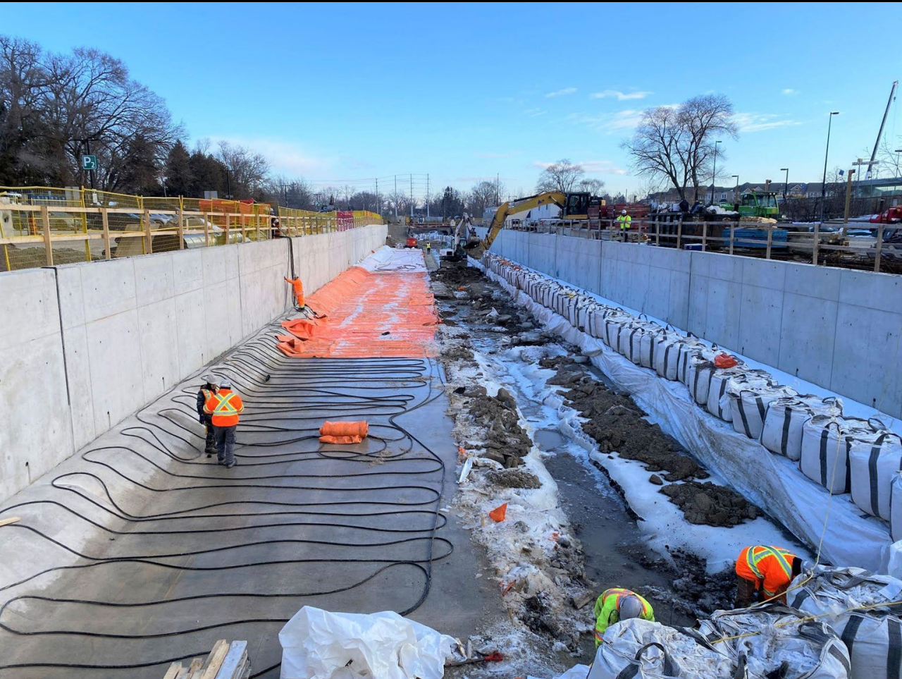
Mary Fix Creek - Channel Excavation
