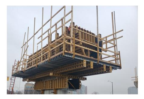
The work in Mississauga Centre has been concentrated between Square One Drive and Eglinton Avenue. Crews are currently busy installing the elevated guideway supported by piers. The placement of girders has begun and will continue into the new year (2023). Once complete the guideway will connect the Hurontario LRT to the MiWay Transit Terminal on Rathburn and facilitate transit users' access to a number of MiWay routes.
