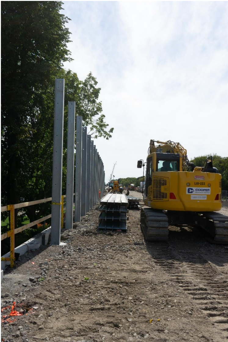
Noise barrier installation
